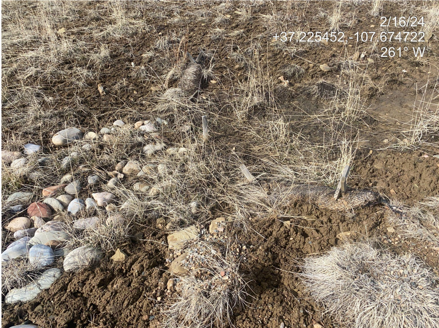
Photo 4. View of wattles in the western interim reclamation area that are not longer functioning.
