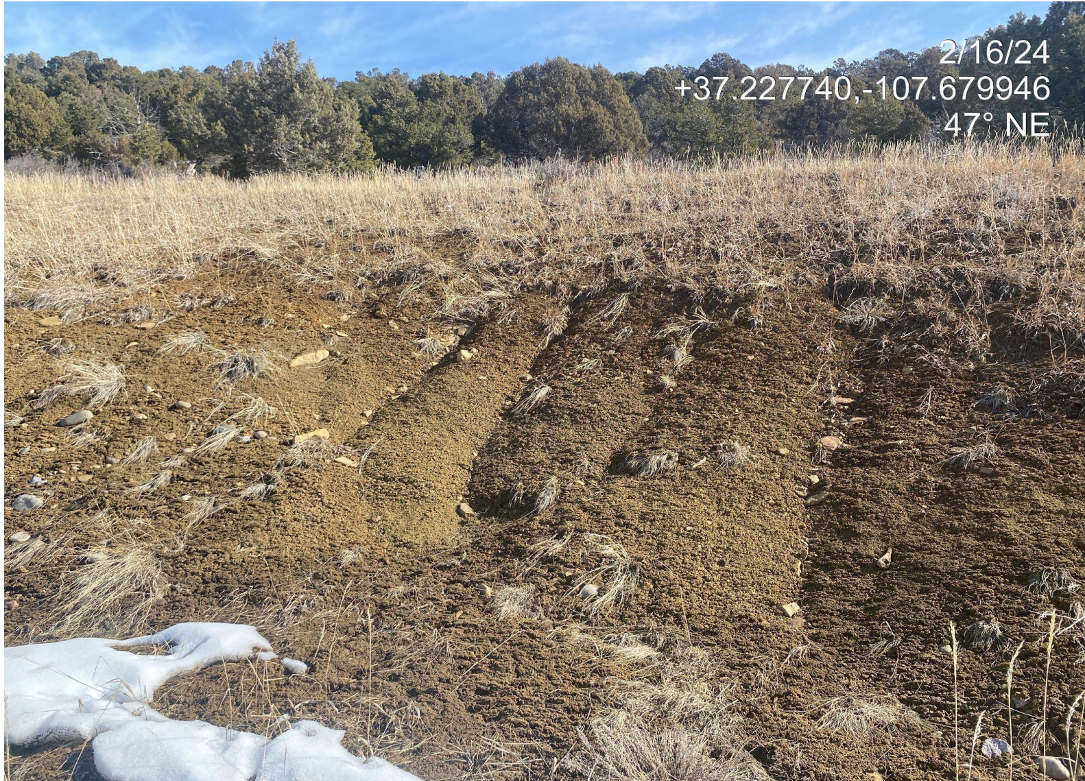
Photo 4. View of rill erosion forming in the northern interim reclamation.
