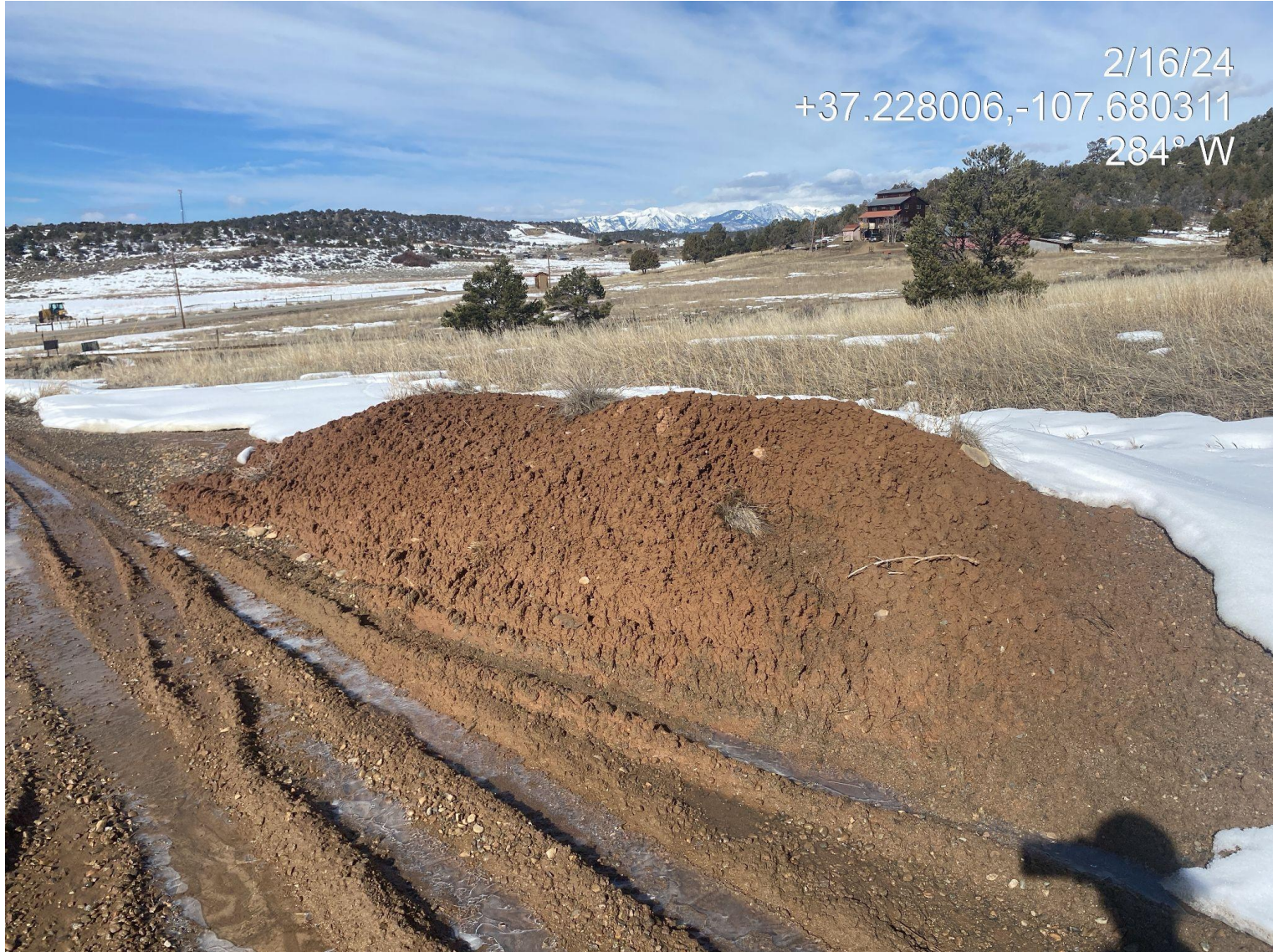
Photo 5. View of exposed/loose soil pile stored on the western edge of the disturbance.
