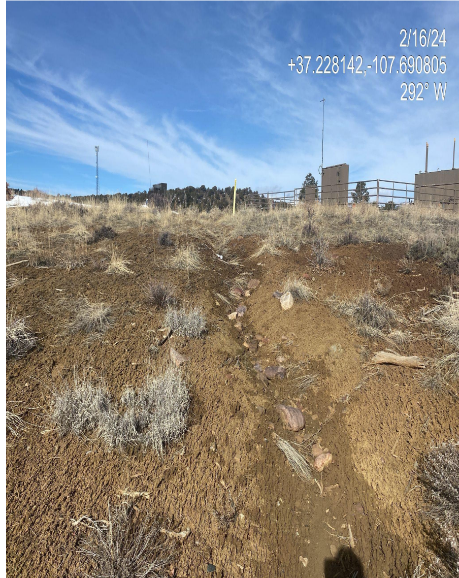
Photo 4. View of rill erosion forming in the southeast interim reclamation area.
