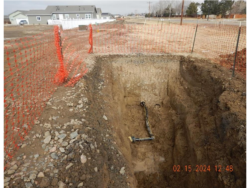
Fenced excavation at south flowline bellhole; 3" HDPE flowline turns west in the excavation. View looking North.
