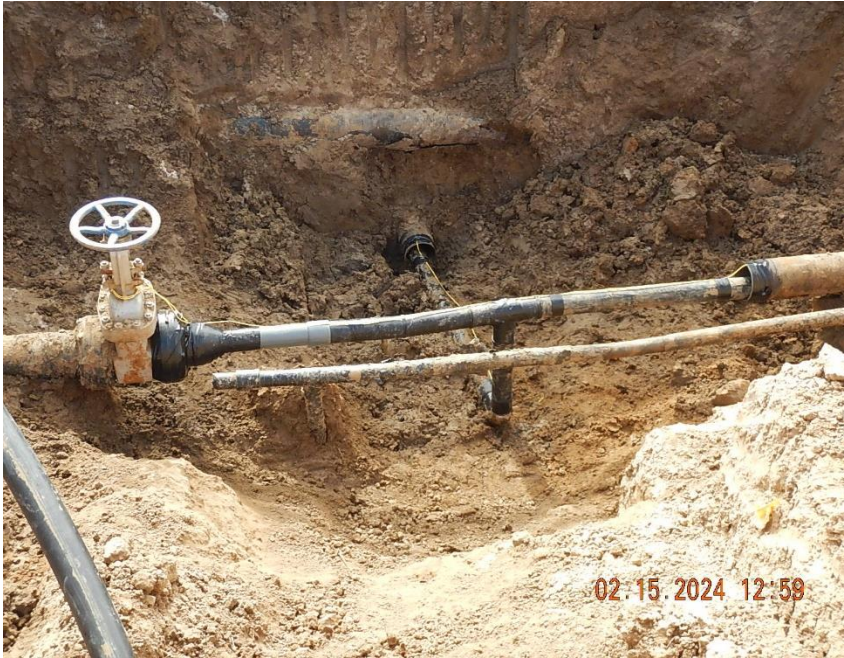
Closer view of flowline repair completed. The existing 6" CS facility #4 flowline transitions to 3" HDPE pipe in both a south and west direction via T fitting/ sliplining. An isolation valve is also present in the excavation.
