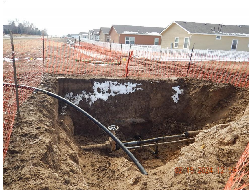
Fenced excavation north of flowline release. Flowline repair pipe (HDPE) and existing consolidation lines are exposed. View looking south on west side of Ridgeway Bd.
