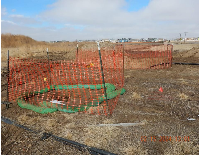
Fenced hydro excavation at spill id #485940 Note: Compromised section of Facility 4 pipe is not exposed
