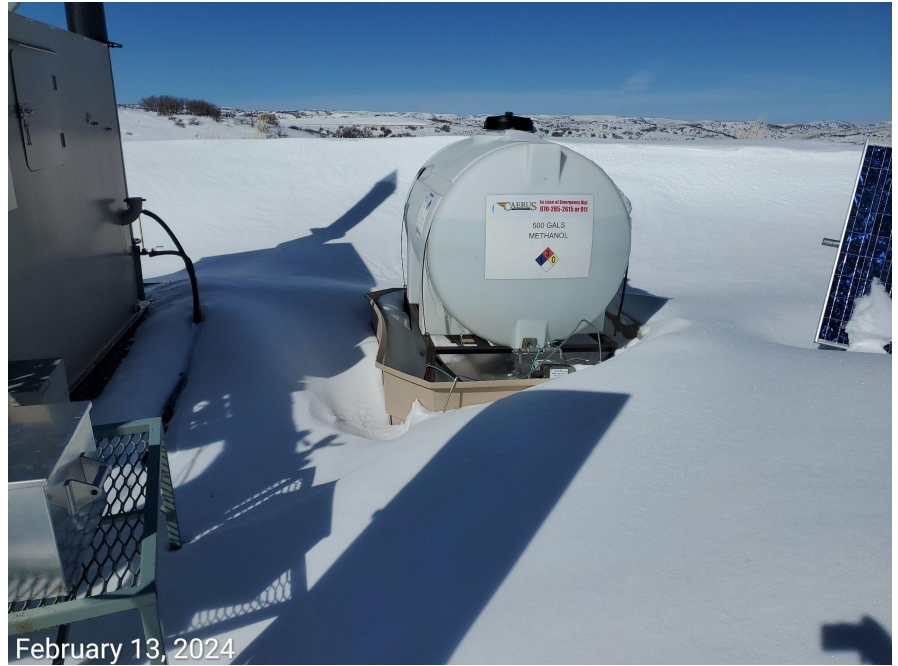
Photo 3: Wildlife protection BMPs missing from the secondary containment of the two methanol tanks on the Location
