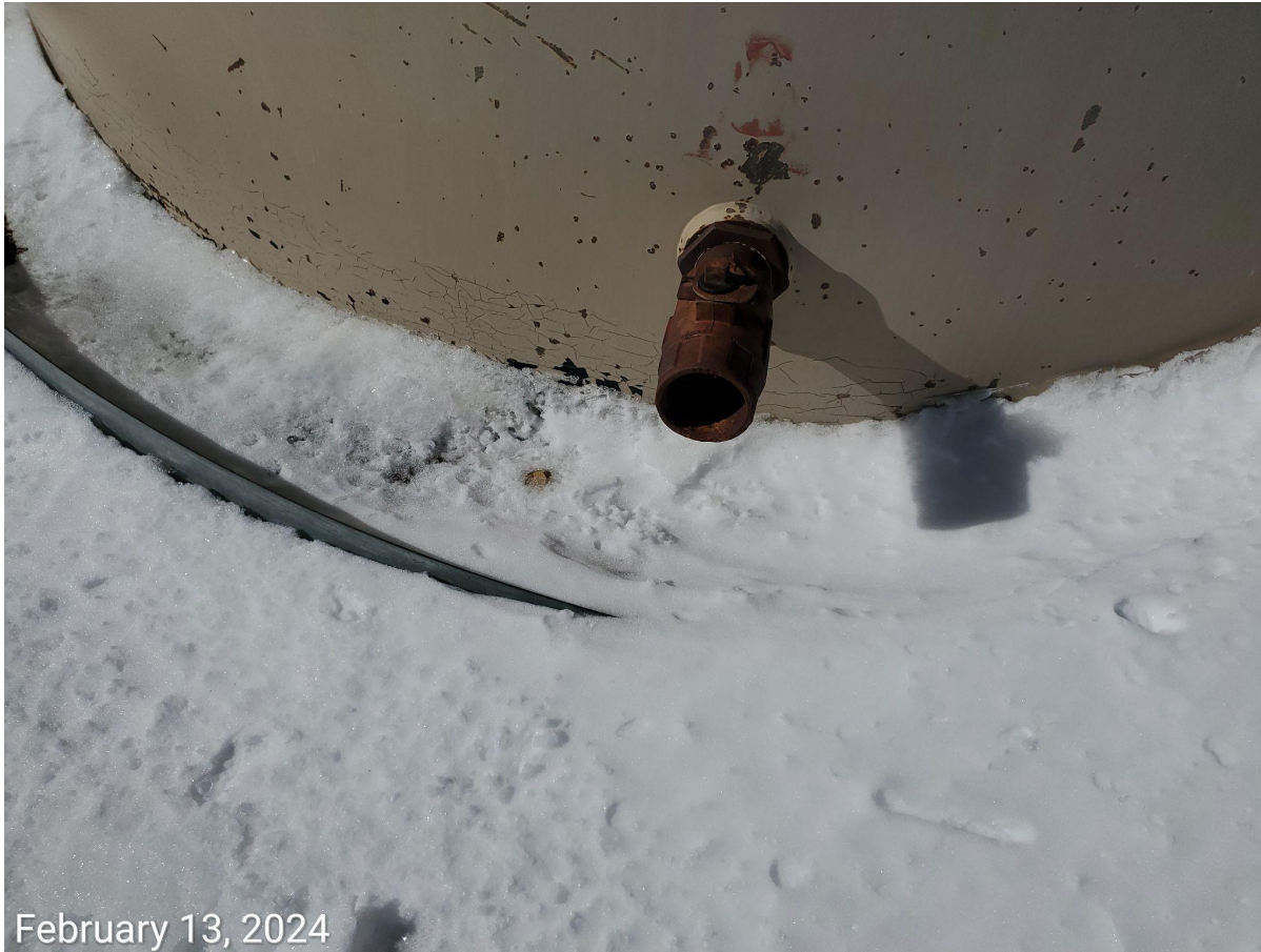
Photo 3: Line at tank missing cap/plug.
