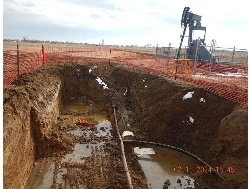
Fenced excavation at flowline release; flowlines exposed. View looking south.
