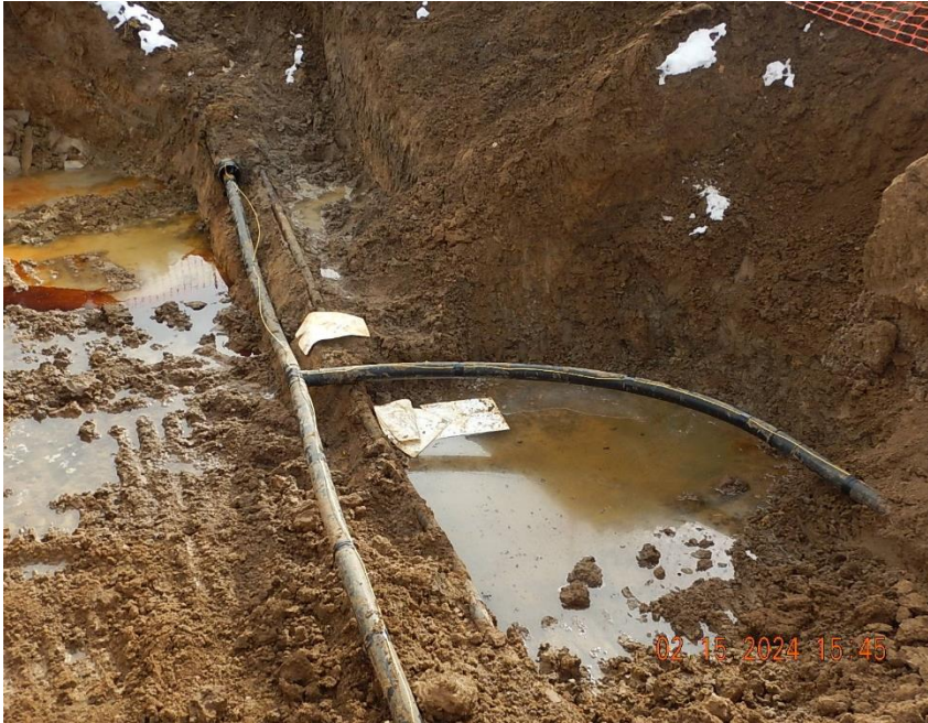
(2) HDPE flowlines with tracer wire installed; sliplined to south through cut/ existing 6" facility 4 carbon steel pipe. (1) existing 2" carbon steel natural gas flowline also seen.
