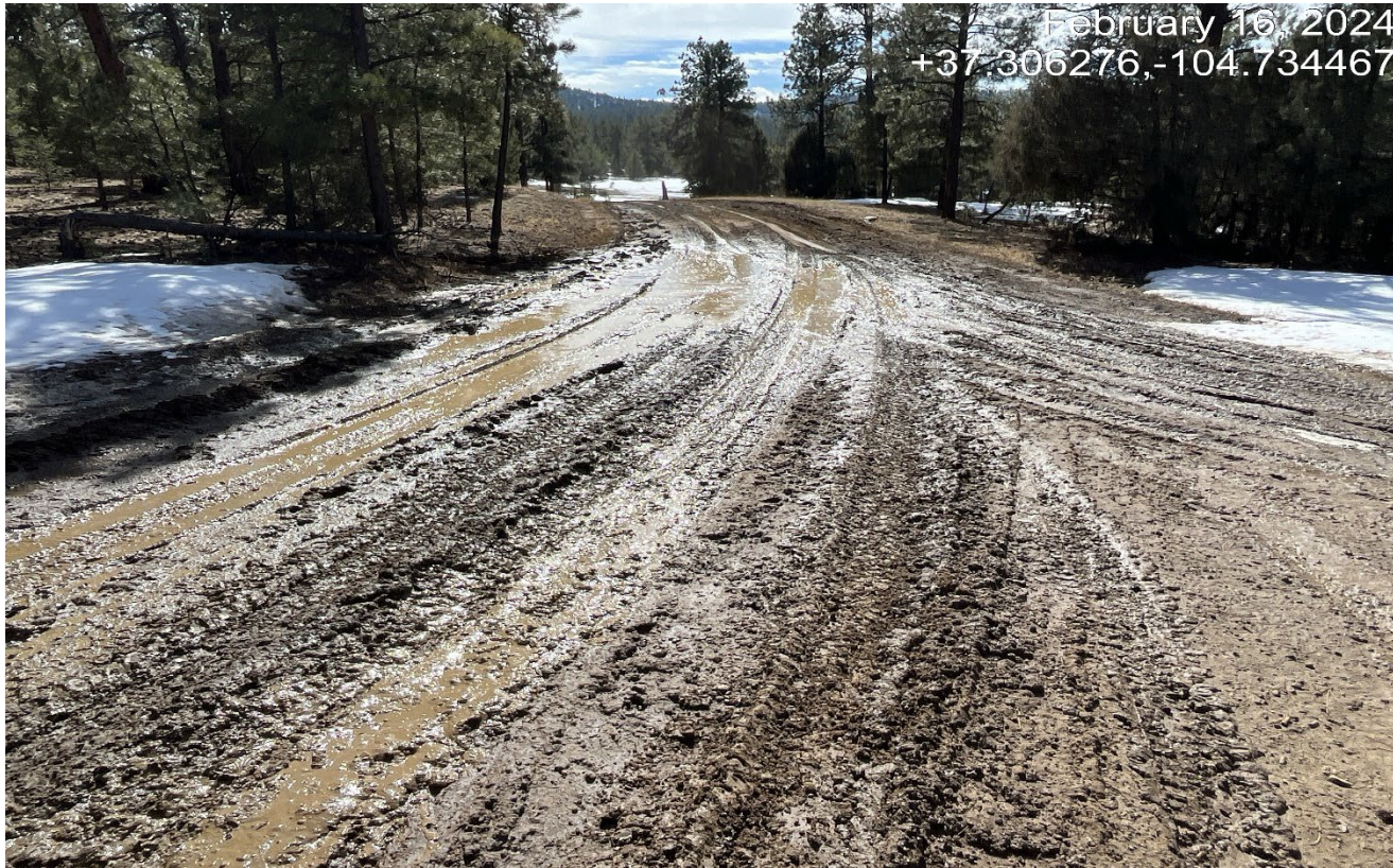
Photo 1. Facing southwest along the access road. There is vehicle rutting and poor drainage along this area.
