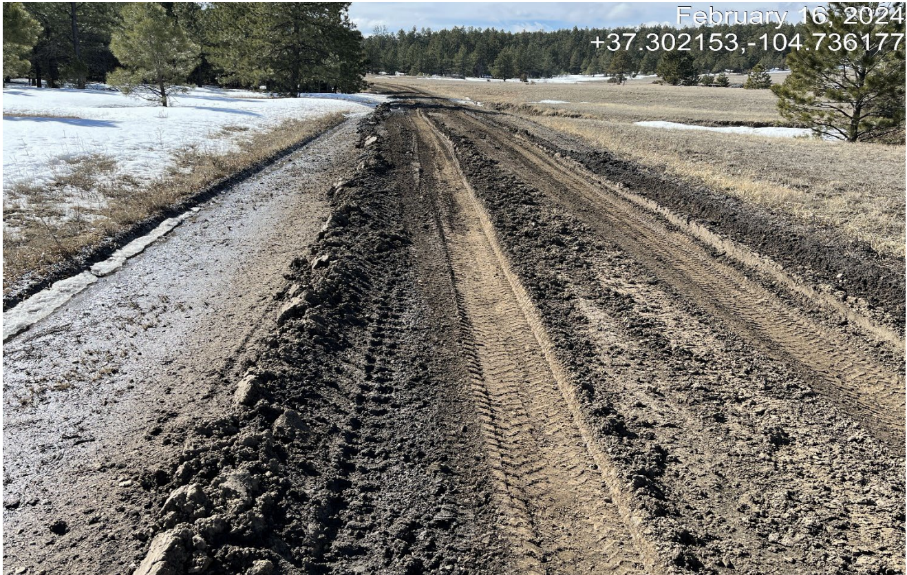
Photo 3. Facing southwest along the access road. There is vehicle rutting along the road which is not stabilized in areas.
