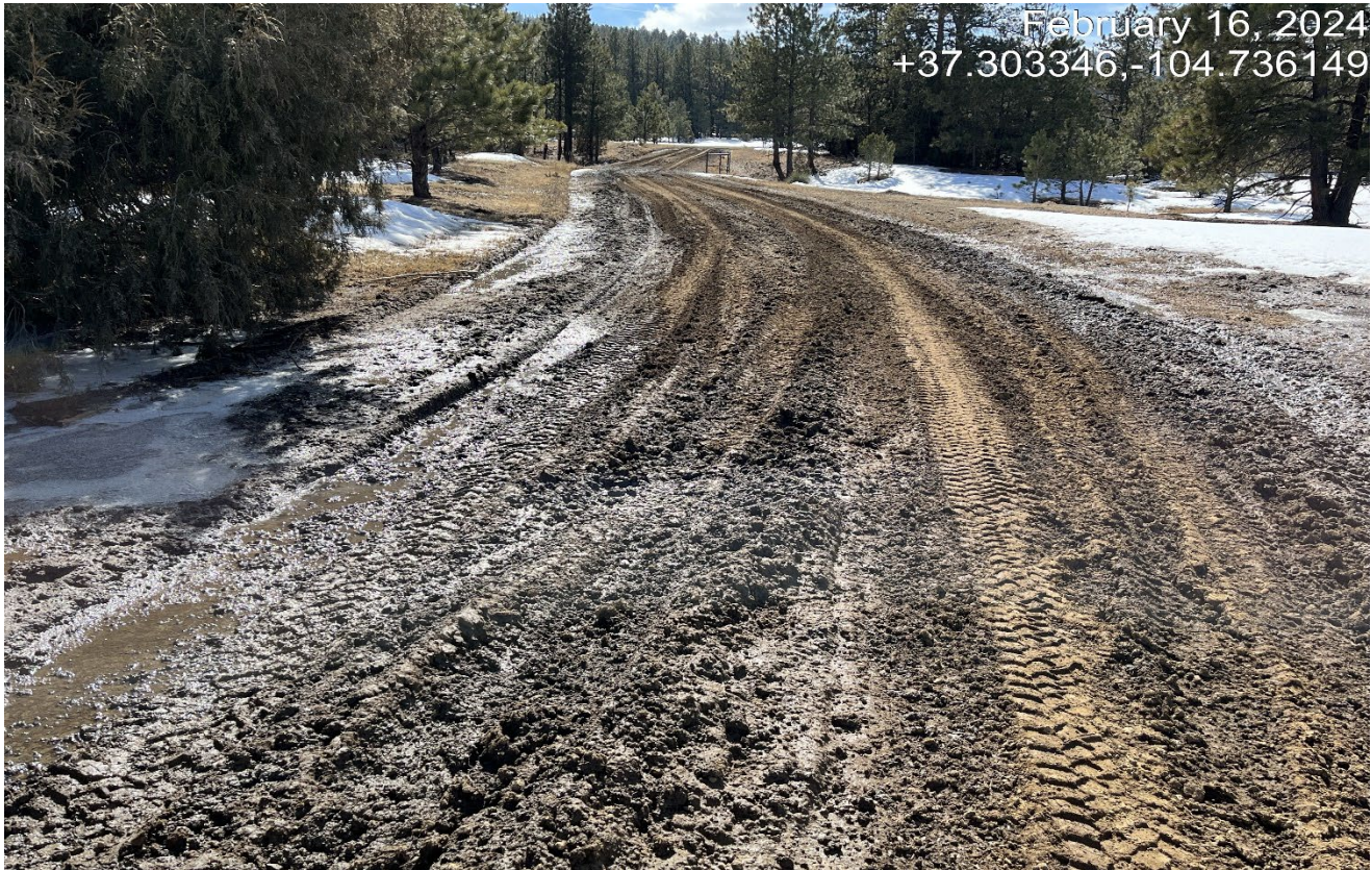
Photo 2. Facing southwest along the access road. There is vehicle rutting and poor drainage along this area.
