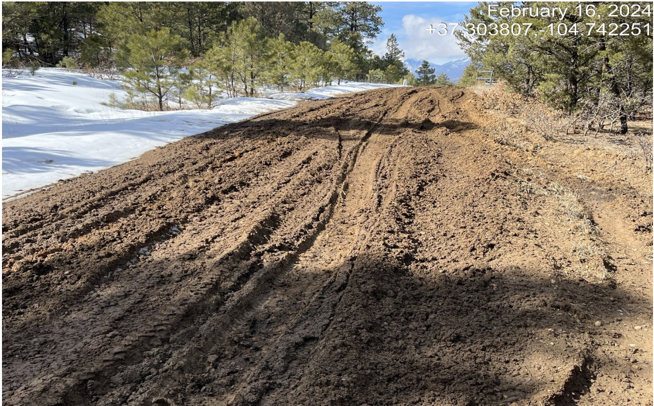
Photo 1. Facing northwest along the access road. There is vehicle rutting and the road is not stabilized along this area.
