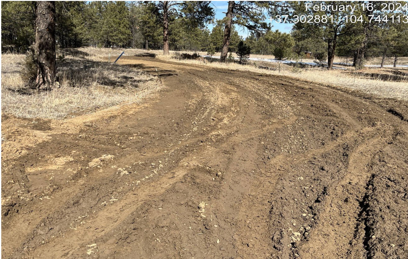
Photo 2. Facing northeast along the access road. There is vehicle rutting and the road is not stabilized along this area.
