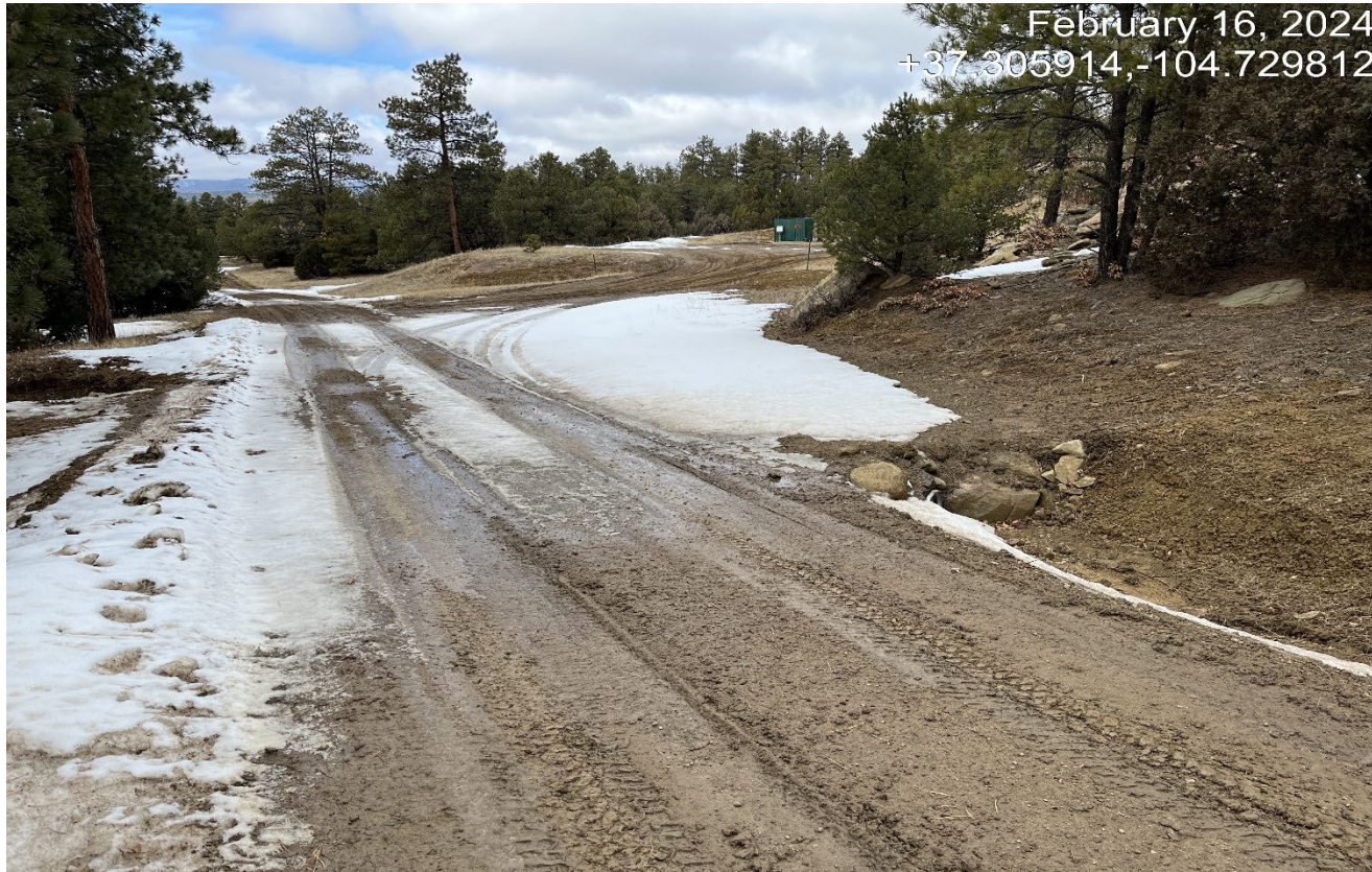
Photo 2. Facing northwest. The culvert near the wellsite has been repaired.
