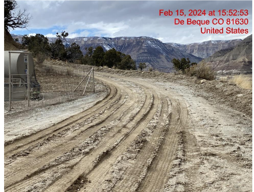
Insufficient Vehicle Tracking BMPs at Location Entrance/Exit – Photo #09332
