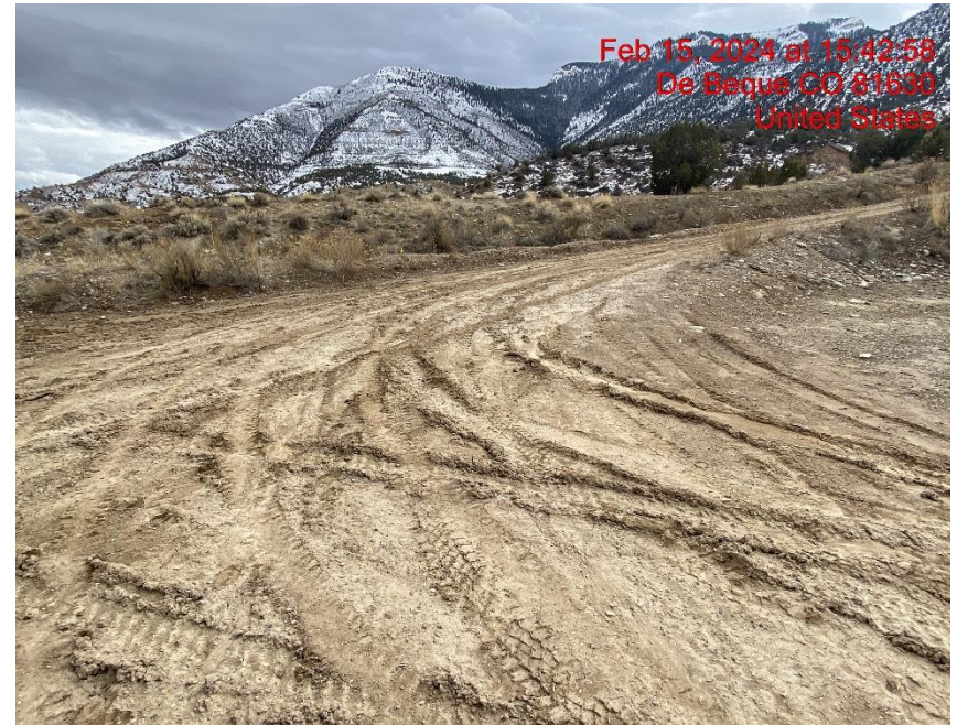
Insufficient Vehicle Tracking BMPs at Location Entrance/Exit – Photo #09325
