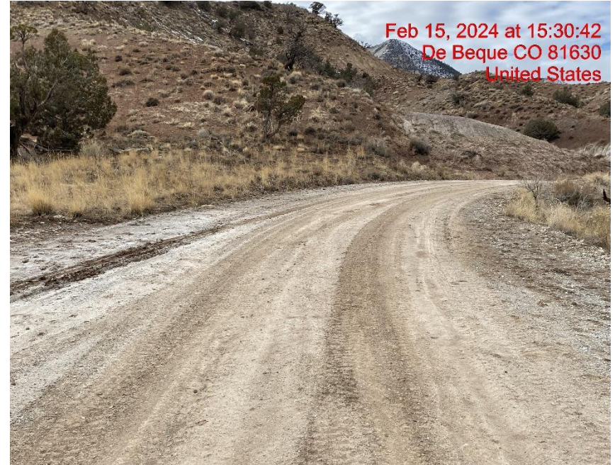
Insufficient Vehicle Tracking BMPs at Location Entrance/Exit – Photo #09316
