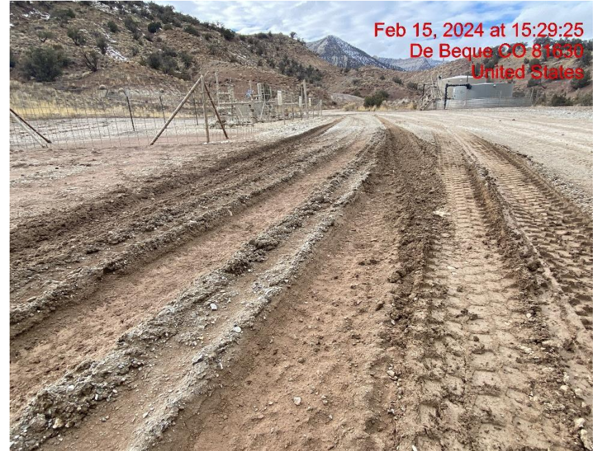
Lack of Stabilization – Photo #09312
