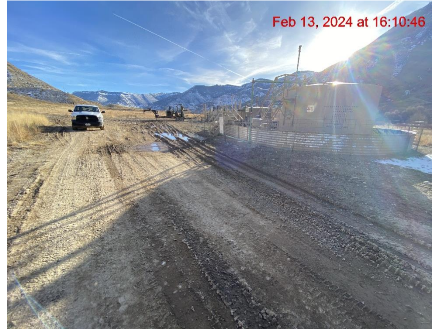
Insufficient Vehicle Tracking BMPs at Location Entrance/Exit – Photo #09298
