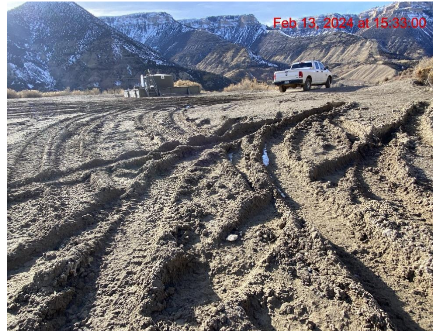
Lack of Stabilization – Photo #09257
