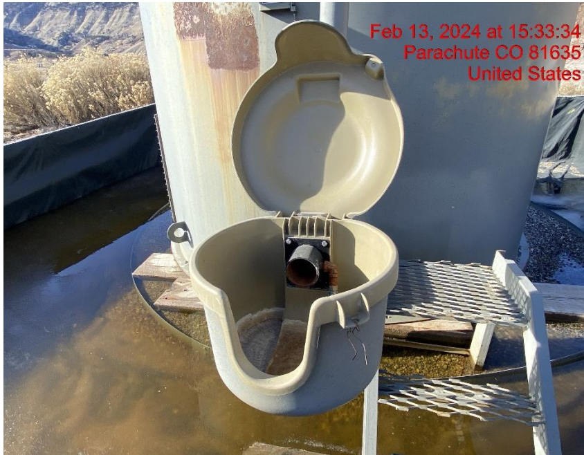
Open-Ended Load Line – Photo #09259
