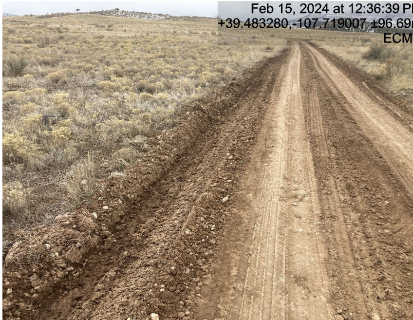
Access road lacking stabilization and trucks driving off side of road
