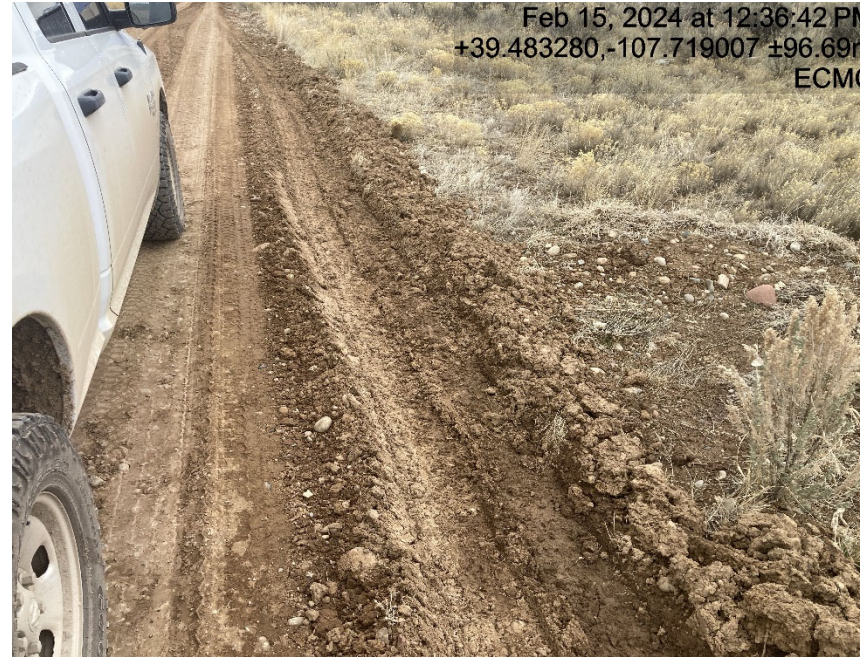
Access road lacking stabilization and trucks driving off side of road
