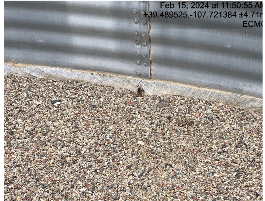
Holes in containment liner
