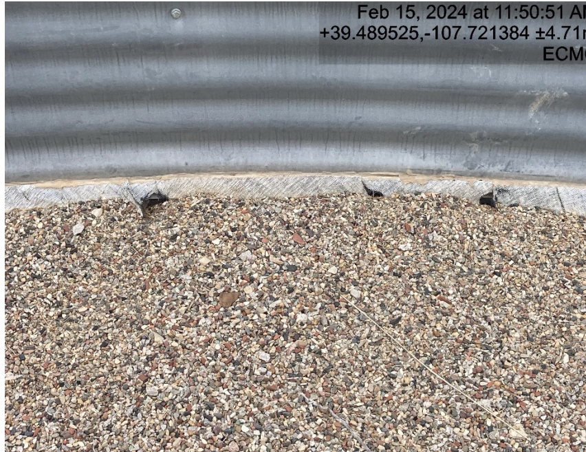
Holes in containment liner
