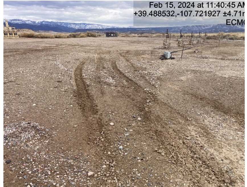
Lack of stabilization/compaction and tracking BMP's
