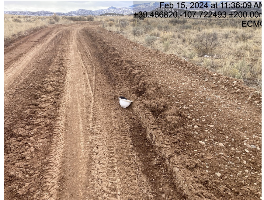
Lack of stabilization/compaction and tracking BMP's
