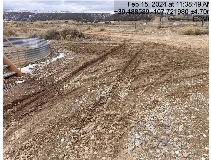
Lack of stabilization/compaction and tracking BMP's
