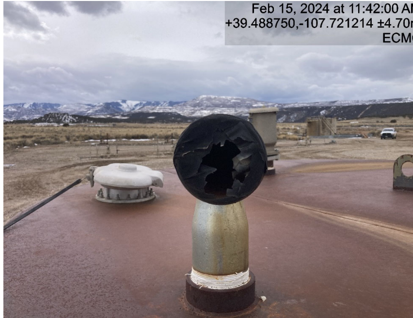
Open pipe on glycol tank
