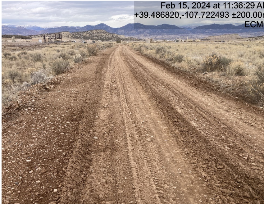
Lack of stabilization/compaction and tracking BMP's
