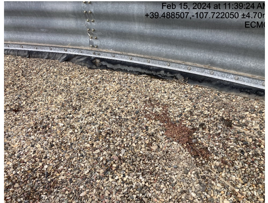
Lining in secondary containment has open holes
