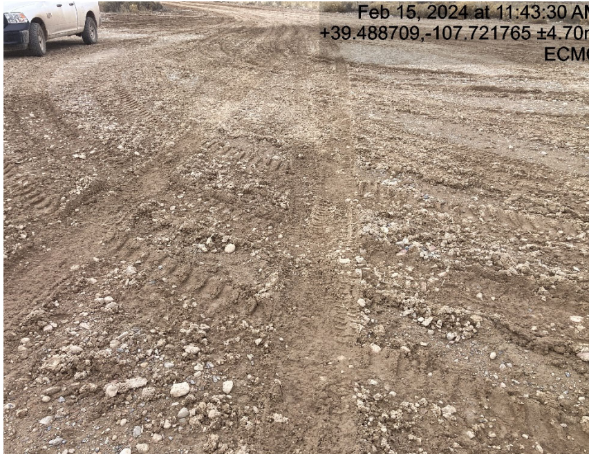
Lack of stabilization/compaction and tracking BMP's
