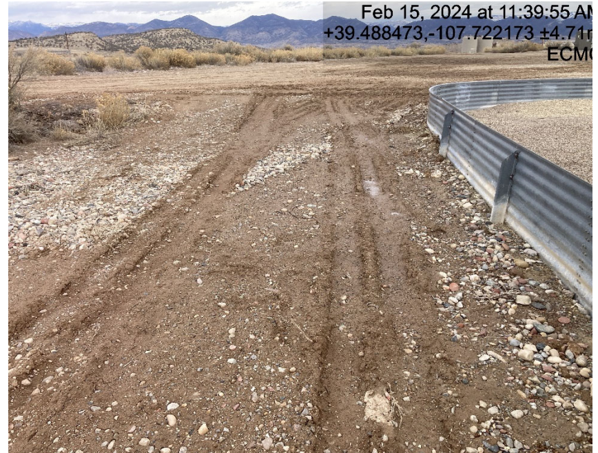
Lack of stabilization/compaction and tracking BMP's
