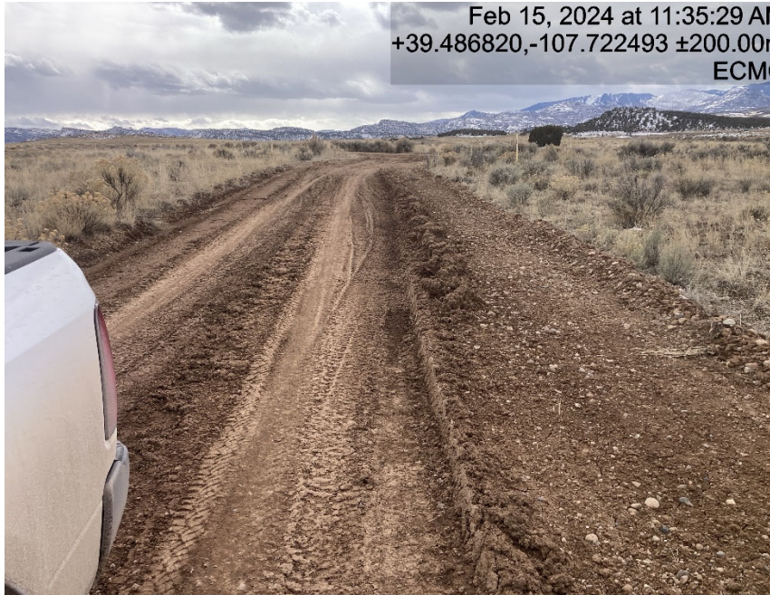
Lack of stabilization/compaction and tracking BMP's
