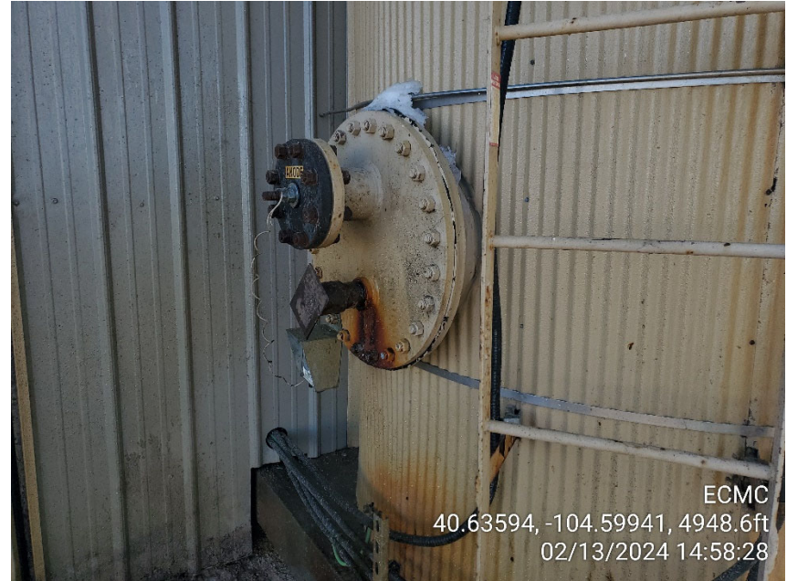
Photo 4 Location of corroded bull plug on heater treater building
