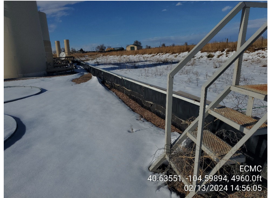
Photo 8 view of liner repair / seam in tank battery containment
