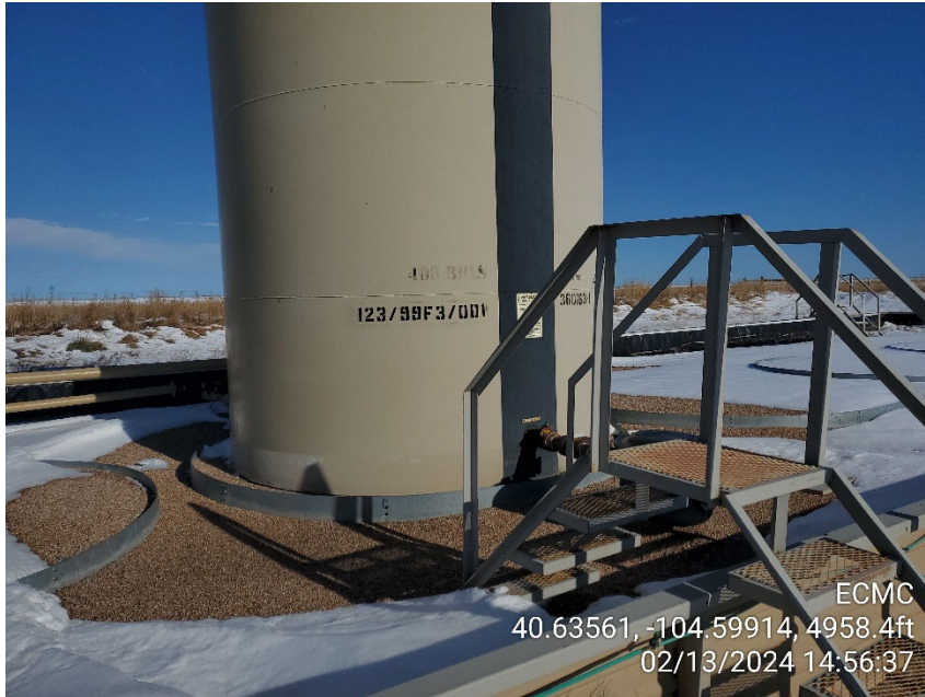
Photo 9 Crude Oil AST, faded labeling
