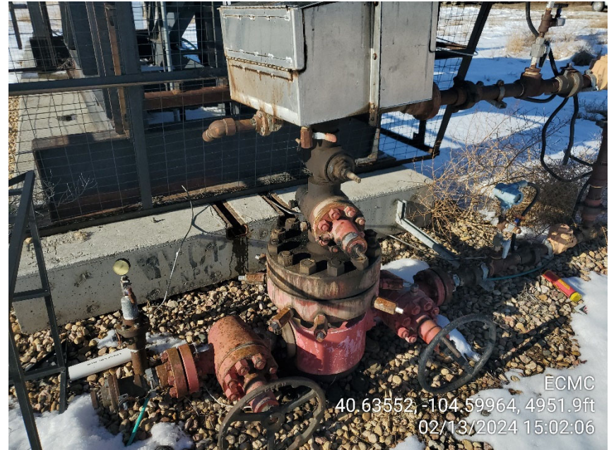
Photo 12 Wellhead, leaky fittings
