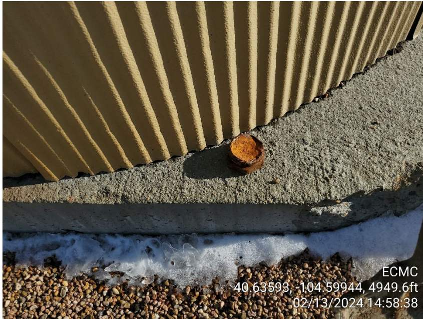
Photo 5 Corroded bull plug
