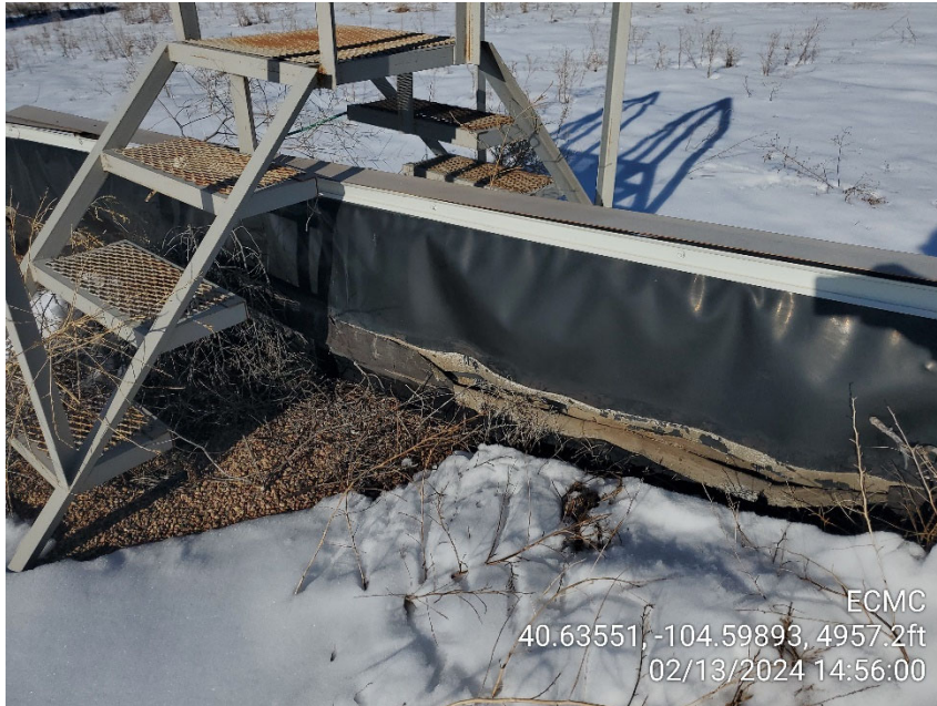
Photo 7 view of liner repair / seam in tank battery containment
