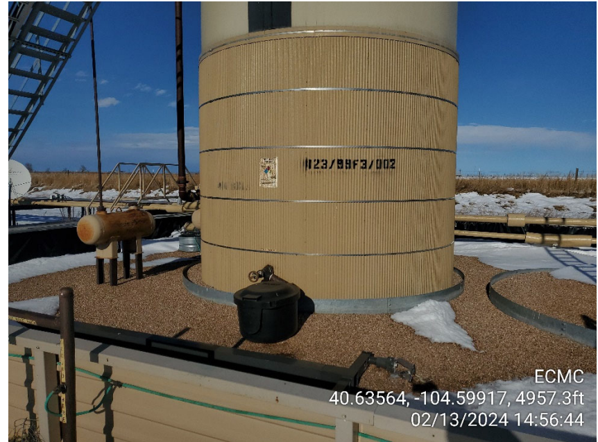
Photo 10 Produced Water AST, faded labeling
