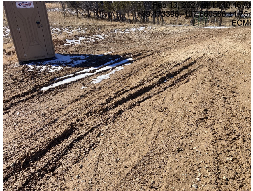
Lacking stabilization/tracking pad
