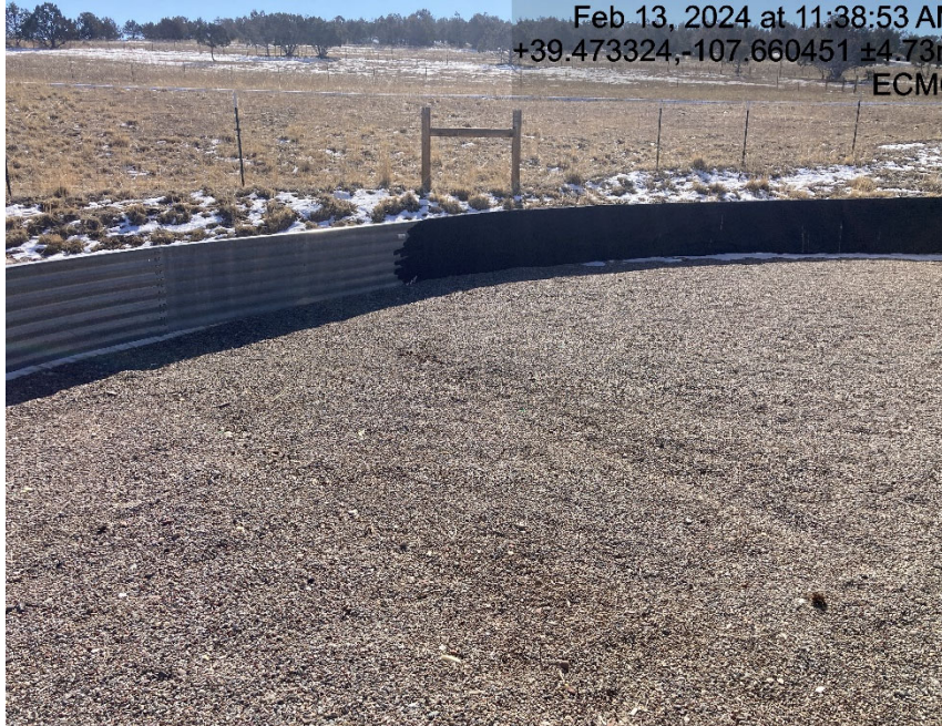
Secondary containment has liner on half of containment?
