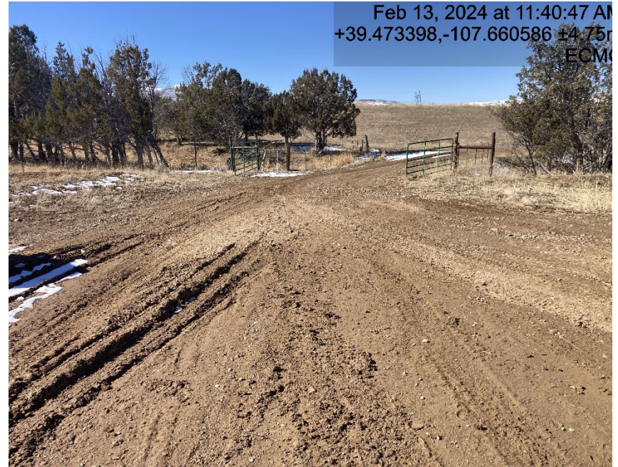
Lacking stabilization/tracking pad
