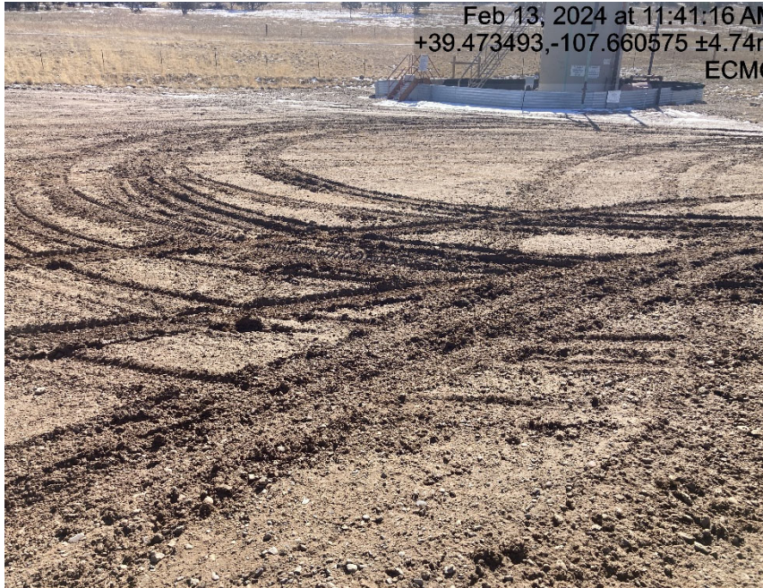
Lacking stabilization/tracking pad
