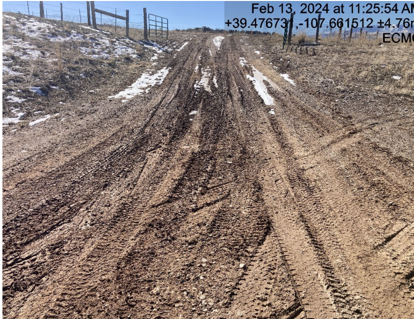
Lacking tracking BMP's and stabilization
