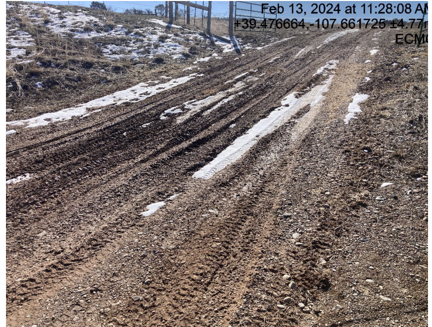
Lacking tracking BMP's and stabilization
