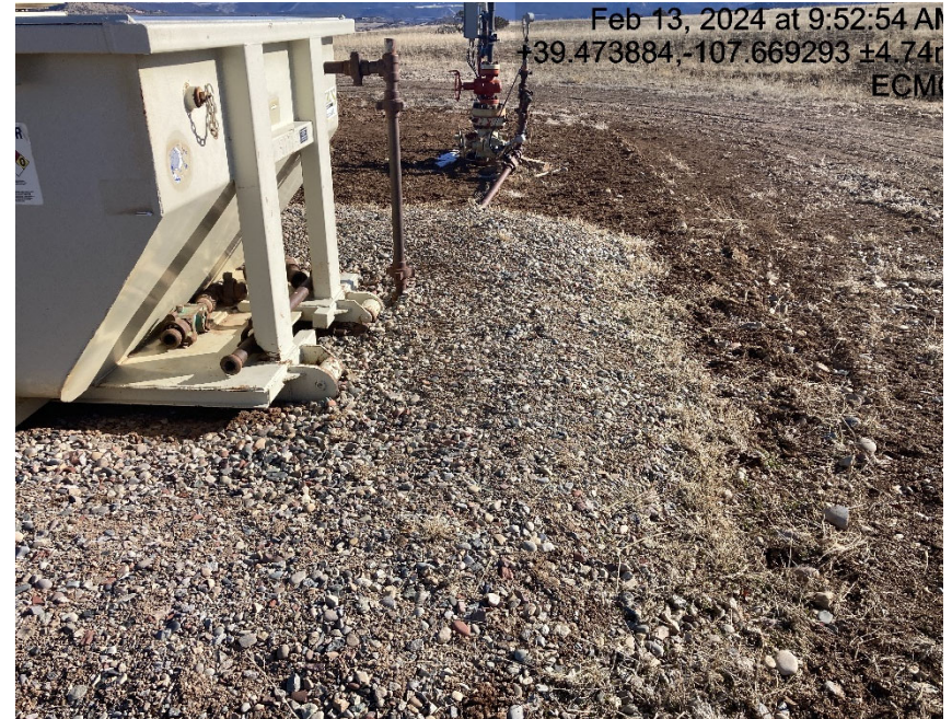
Lacking effective secondary containment
