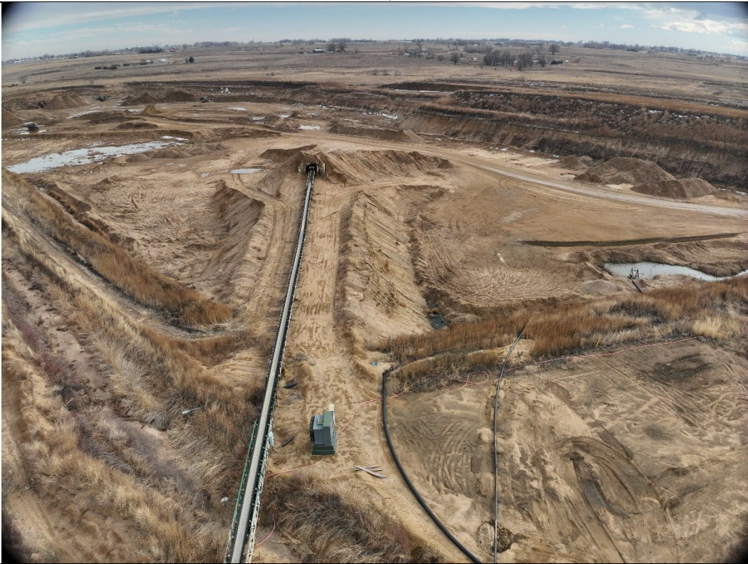
In View – Well Nelson #23-32 (API # 05-123-19599 ), Tank Battery, Flowlines
