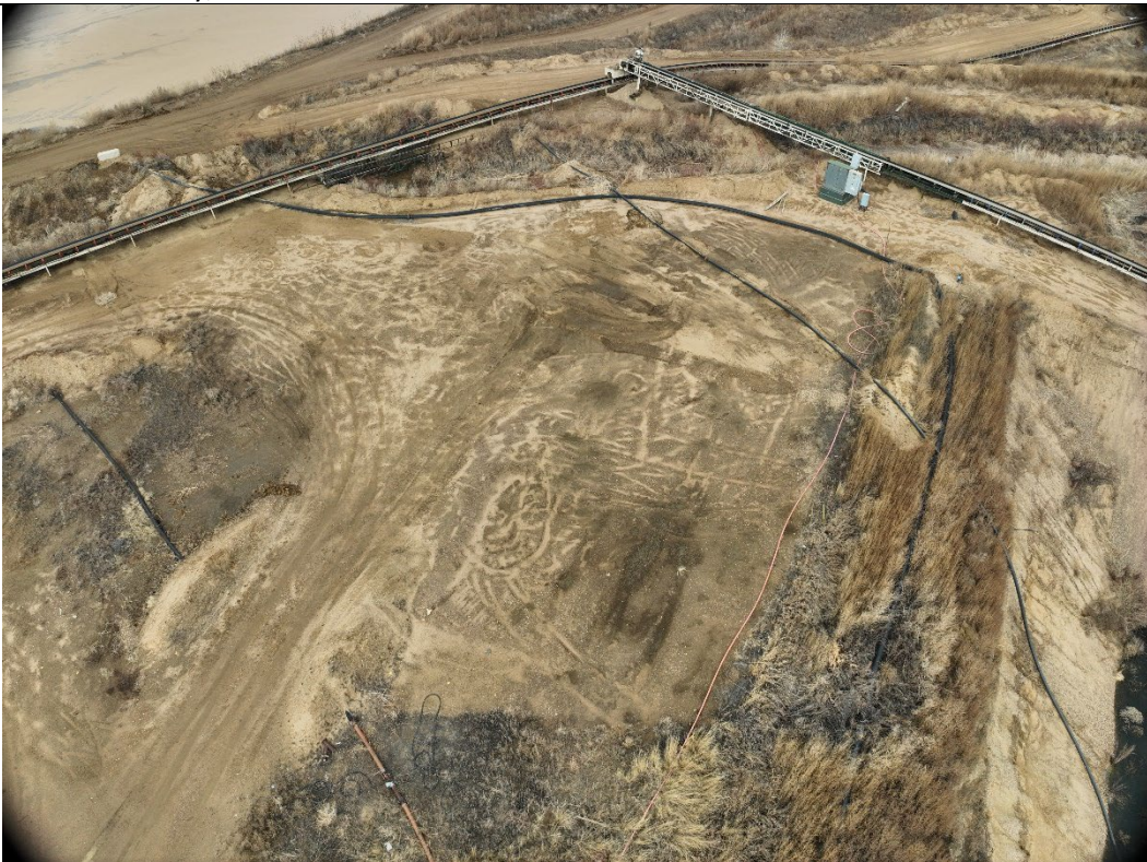
In View – Tank Battery, Flowlines
