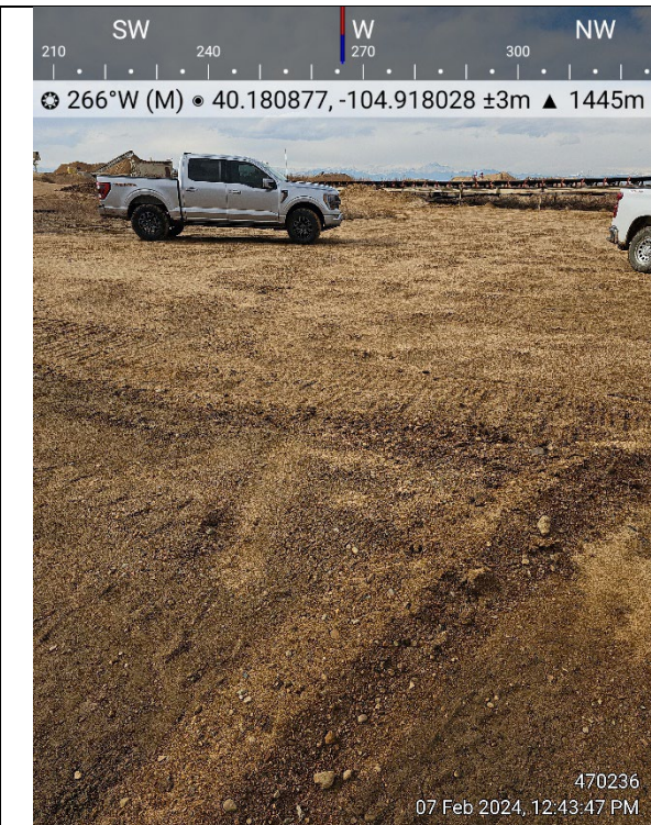
Looking West at tank battery and separator location – 40.180877 / -104.918028
