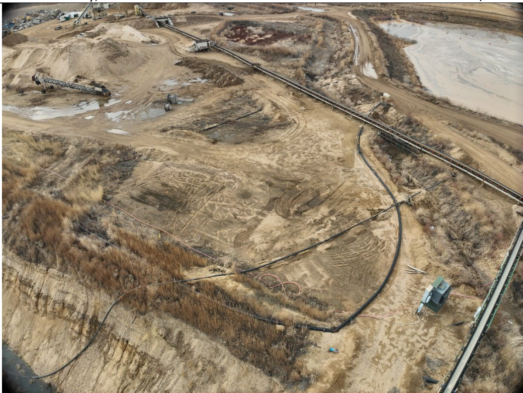
In View – Tank Battery, Flowlines
