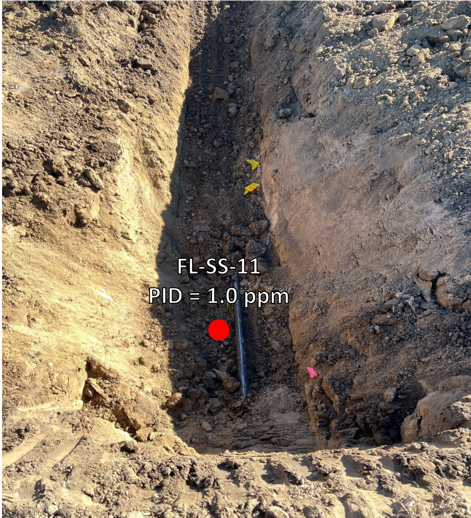
Looking east at bellhole/cut point for removal
