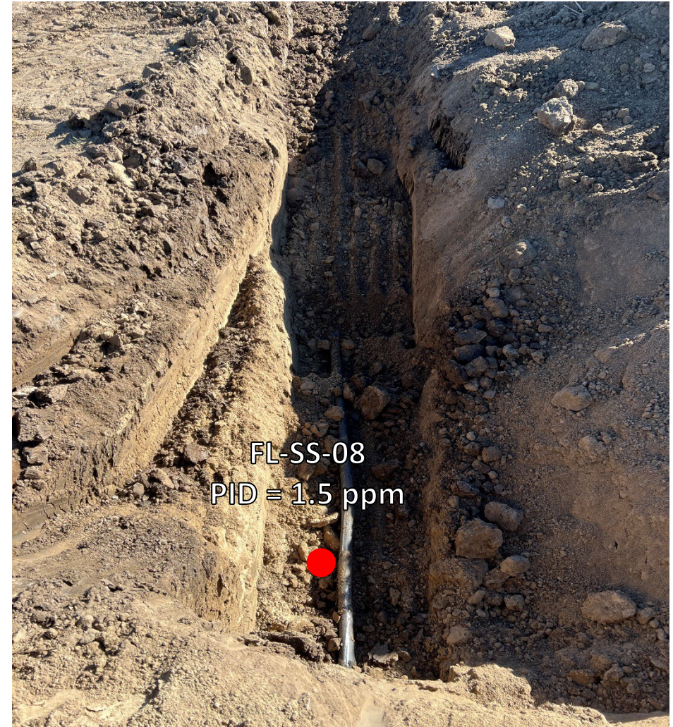
Looking east at bellhole/cut point for removal
