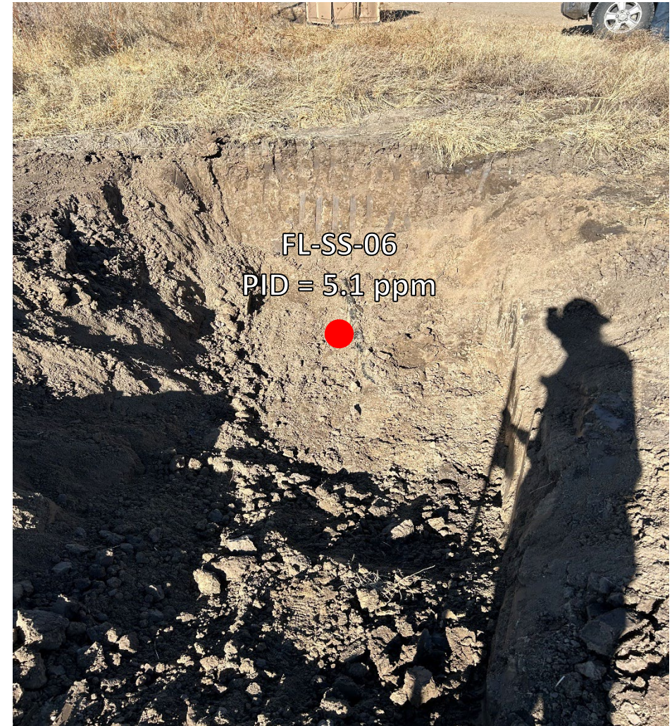
Looking north at flowline directional change
