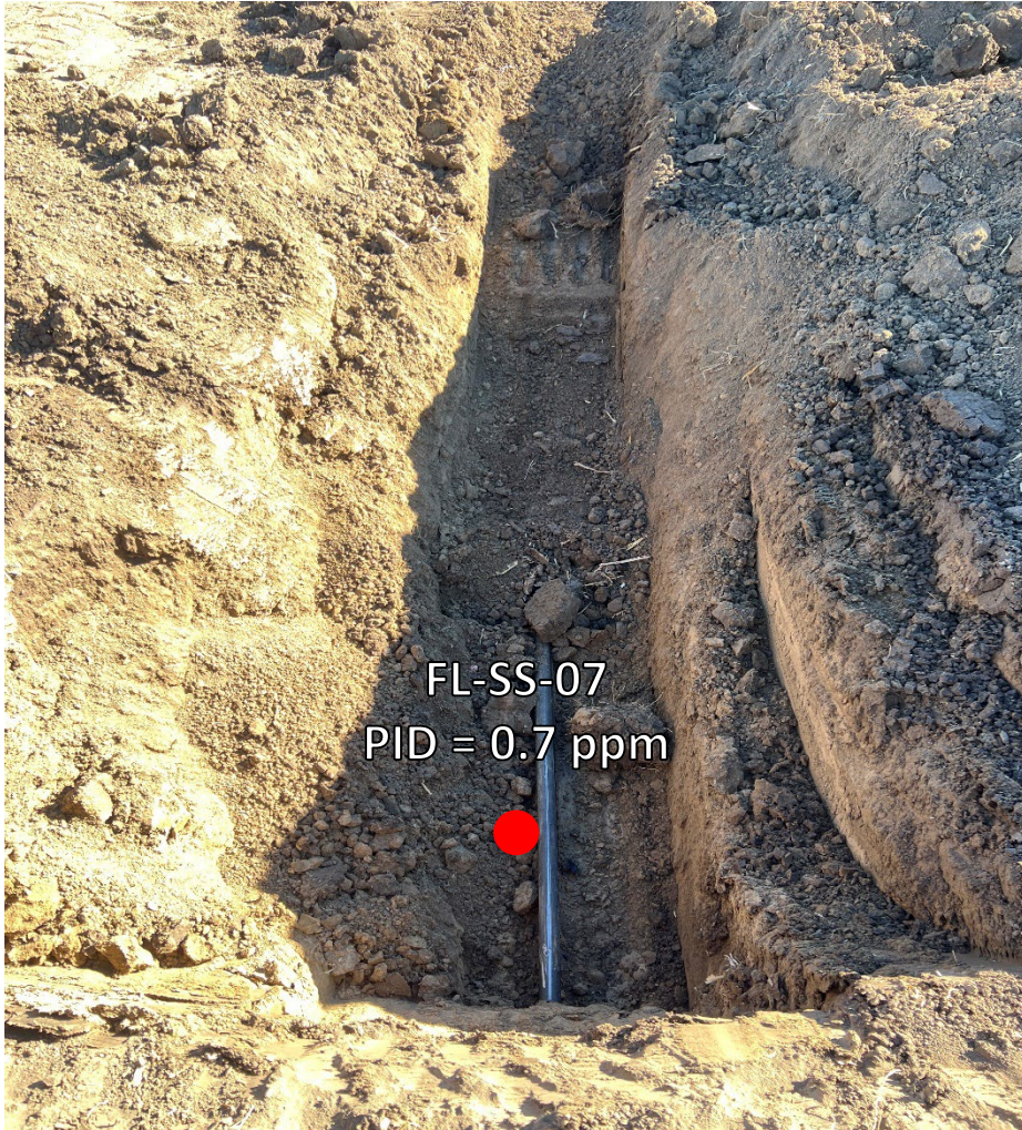
Looking east at bellhole/cut point for removal
