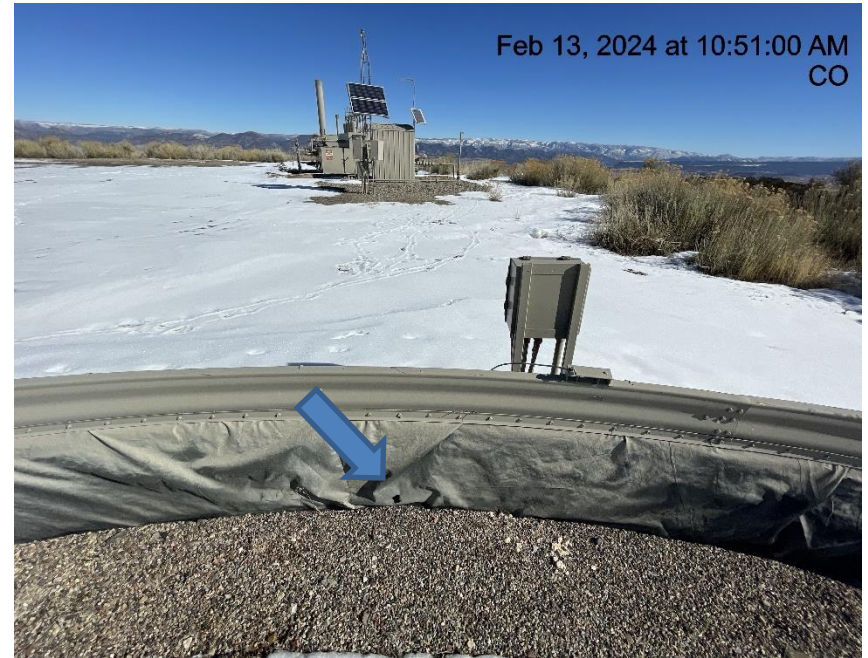
Photo # 6474 Hole in liner/liner needs maintenance
