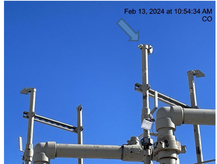
Photo # 6476 Rupture disc vent line lacks cap
