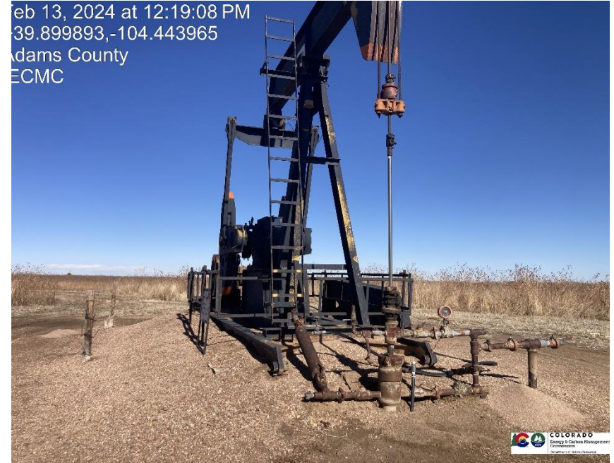
Pic 2 pump jack / wellhead
