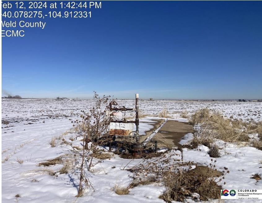
Pic 1 Wellhead / some weed growth
