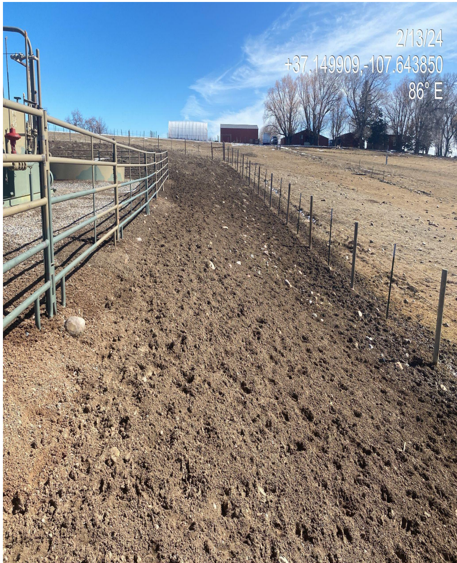
Photo 2. Cut and fill slopes lacking vegetation with exposed soil. Disturbance has been degraded by exposure to cattle in the area, no vegetation establishment in the interim reclamation areas.
