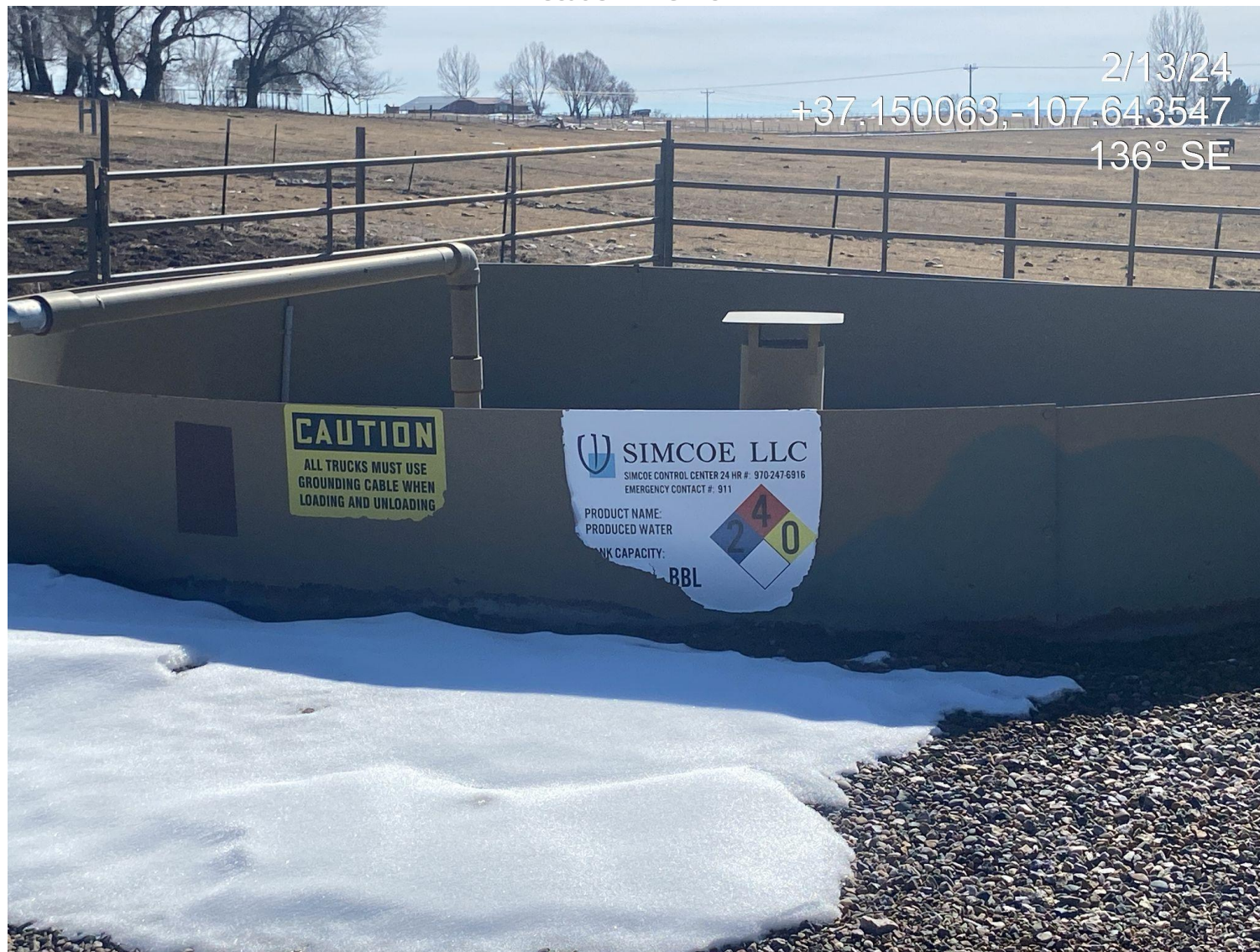
Photo 3. View of deteriorating produced water sign that is no longer displaying max capacity.
