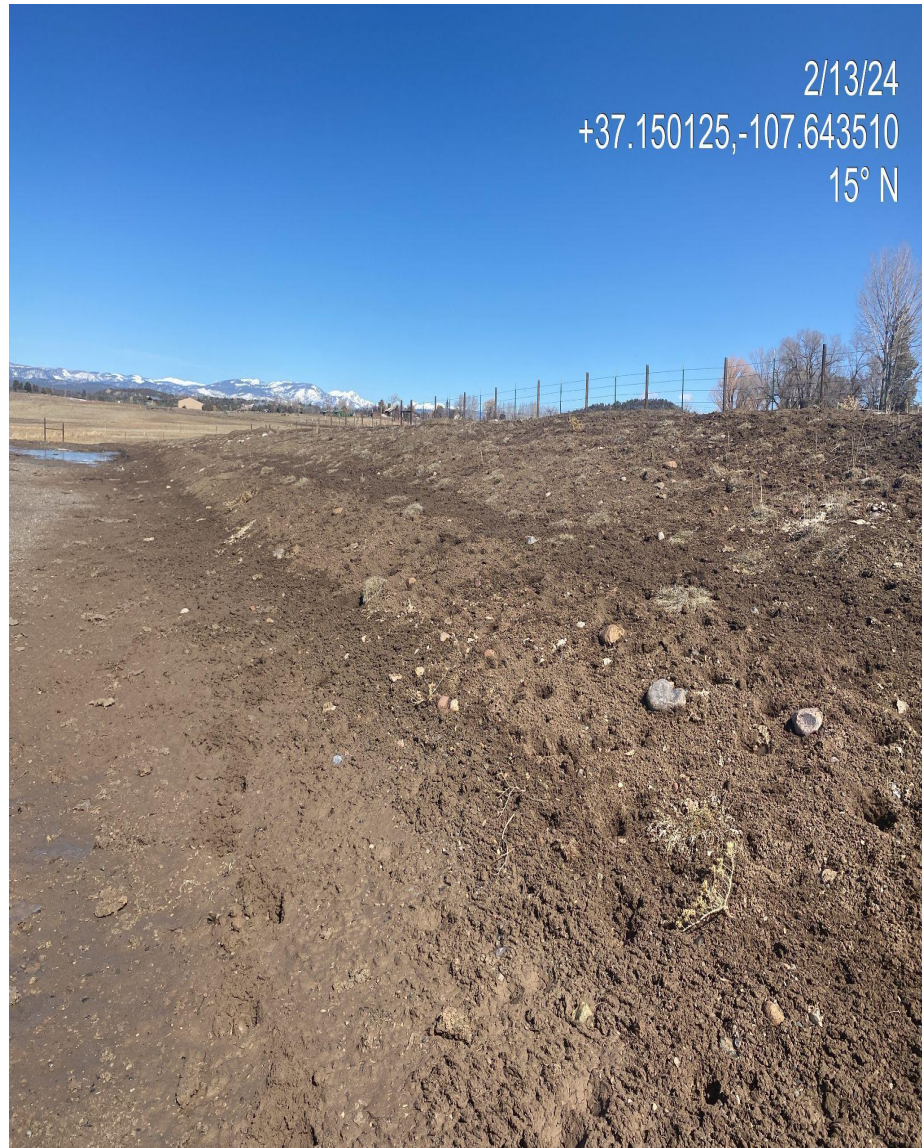
Photo 2. Cut and fill slopes lacking vegetation with exposed soil. Disturbance has been degraded by exposure to cattle in the area, no vegetation establishment in the interim reclamation areas.
