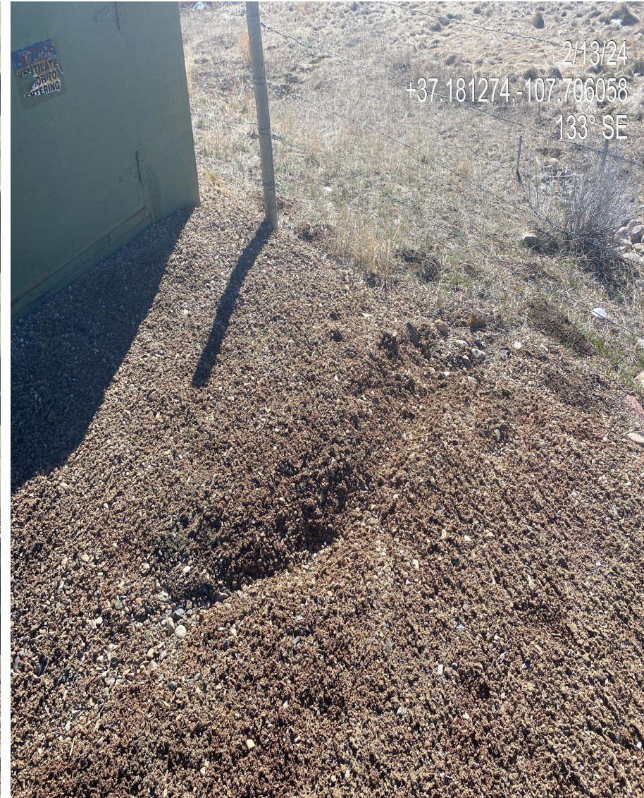
Photo 3. View of rill erosion forming on the southern edge of the disturbance.
