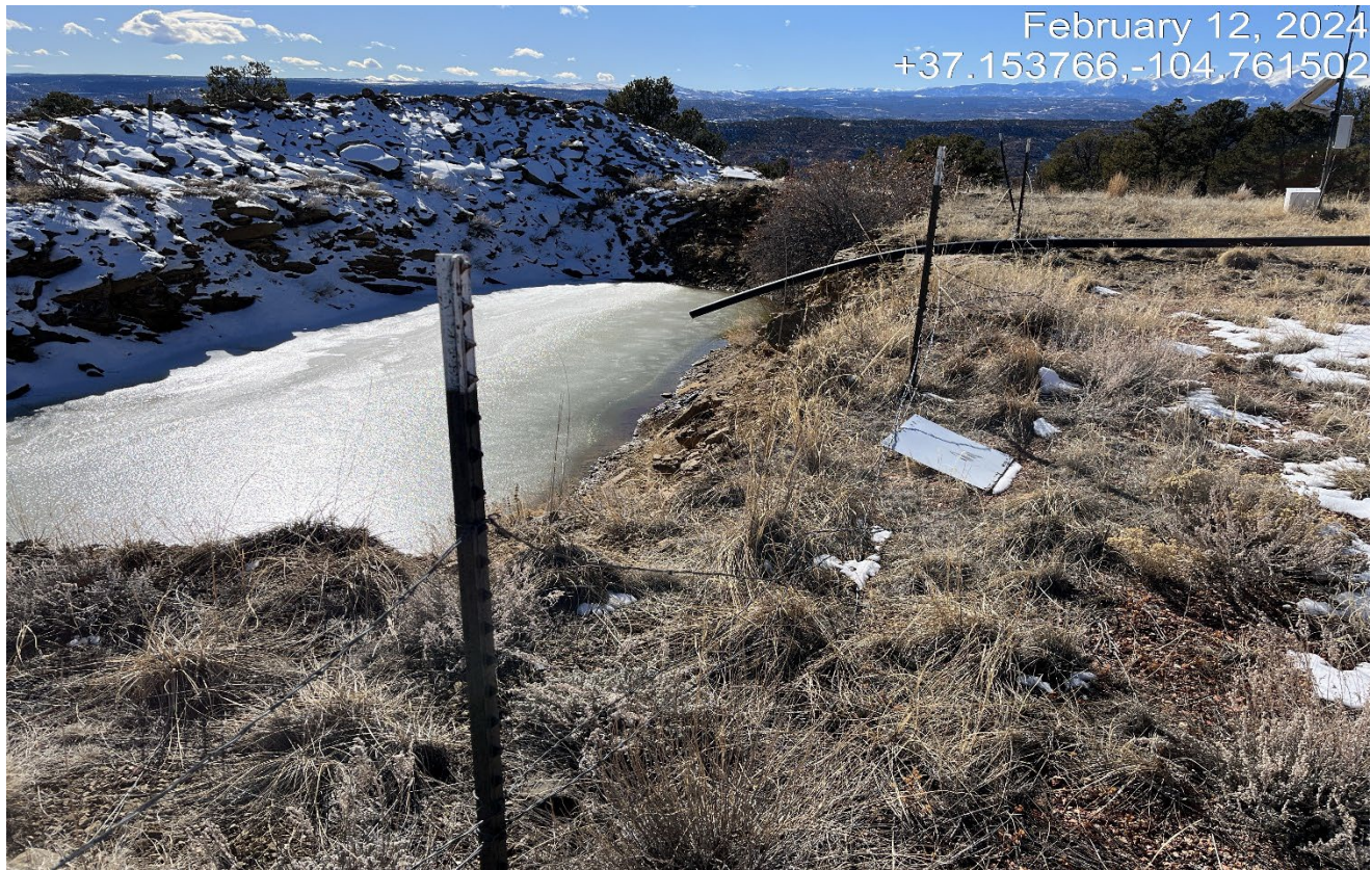
Photo 2. The fence around the pit is in disrepair..
