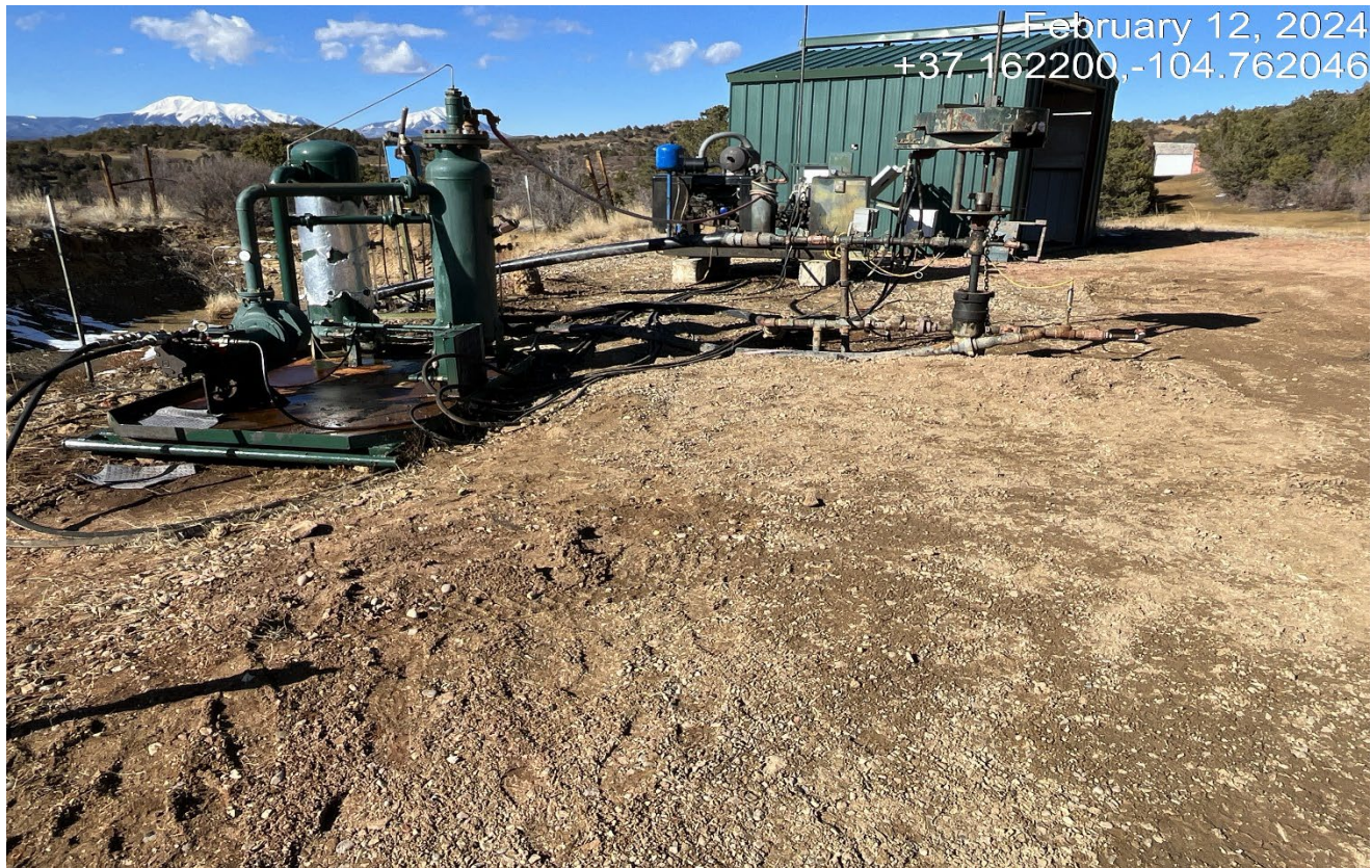
Photo 2. Facing toward the wellhead. There are stained soils at wellhead and separator that need to be cleaned up.
