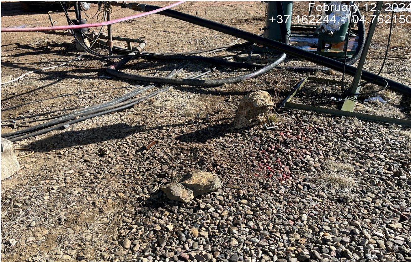
Photo 3. There is stained soils around the wellhead from a recent spill..
