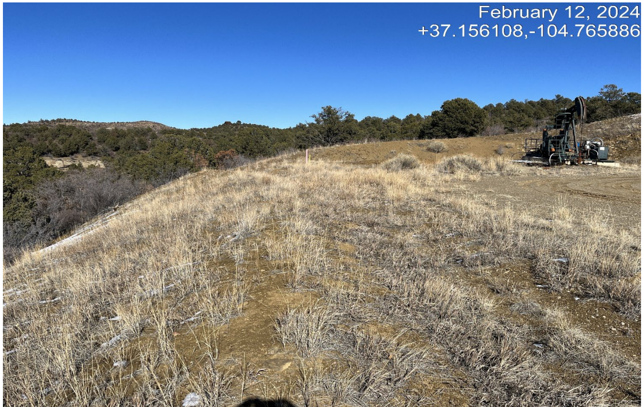
Photo 2. Facing north along the fill slope which is stabilized with vegetation.
