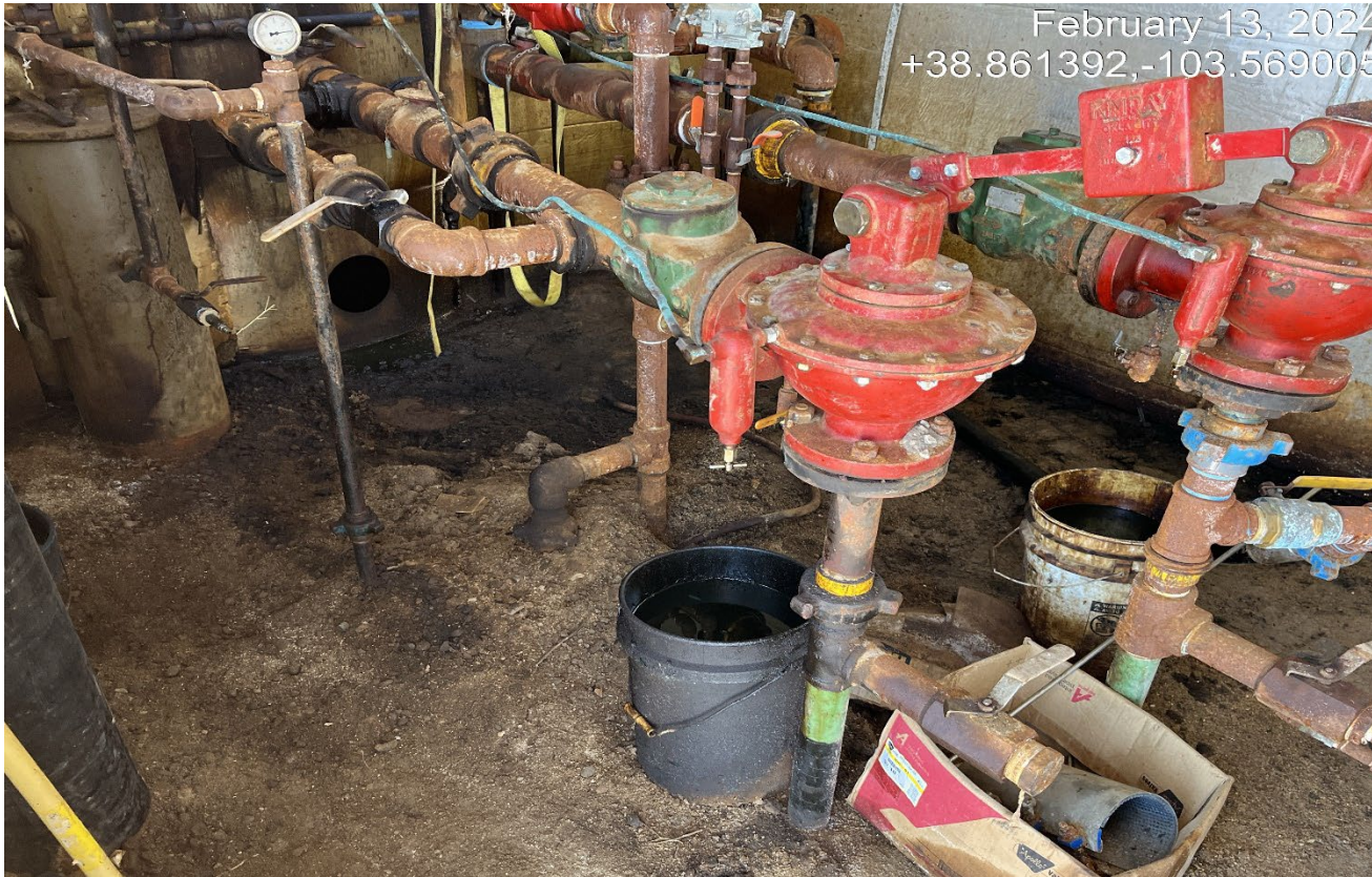
Photo 6. Inside the shed next to the treater. There is oil saturated soils inside the shed. There are full buckets of oil that appear to be collecting oil from leaking pipes.
