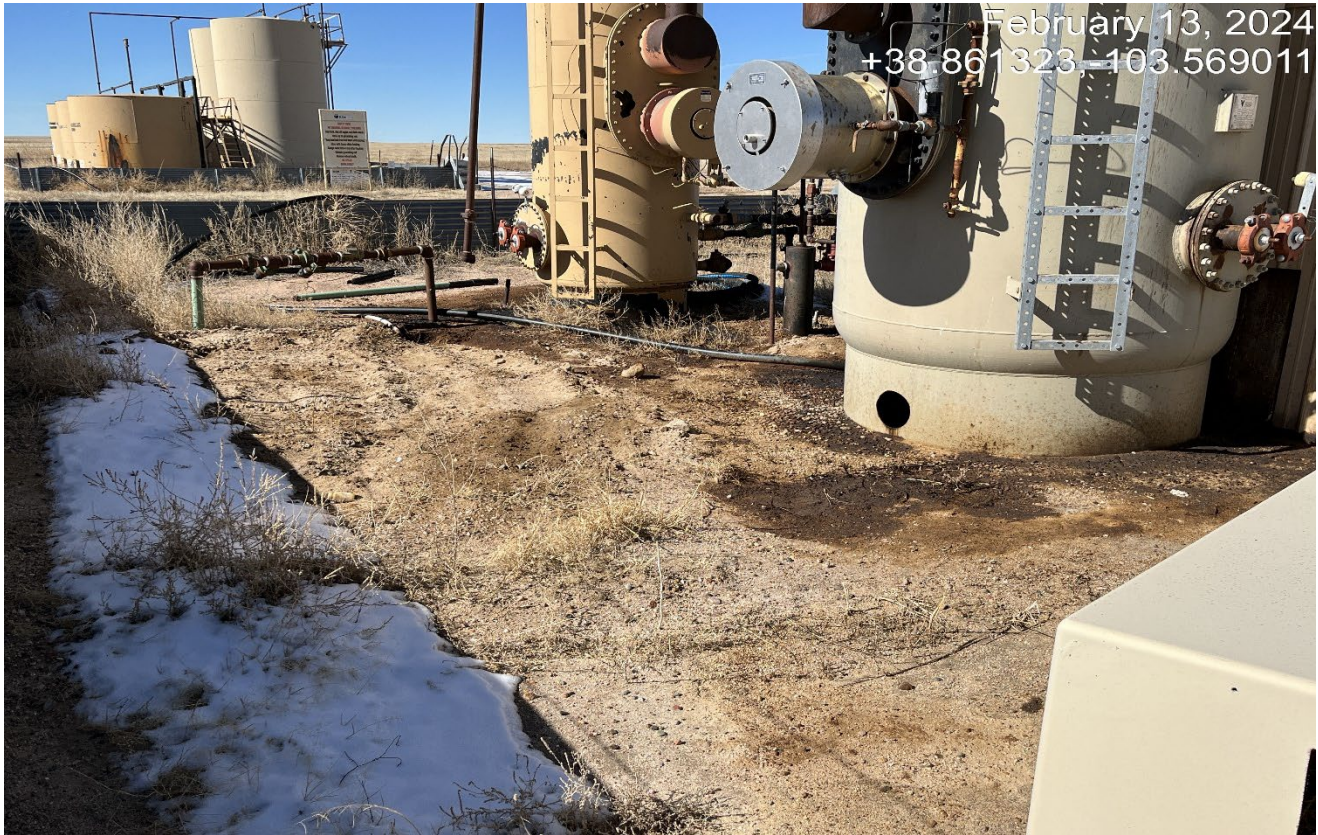
Photo 3. Facing toward the backside of the treater. There has been oil leaked out onto the ground that must be cleaned up.
