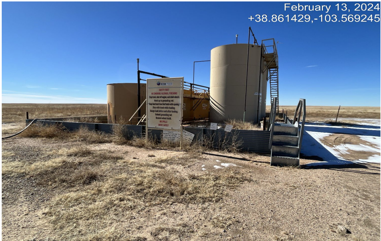
Photo 7. Facing toward the tank battery at the southwest side. There is some weed debris inside the containment that needs to be removed.
