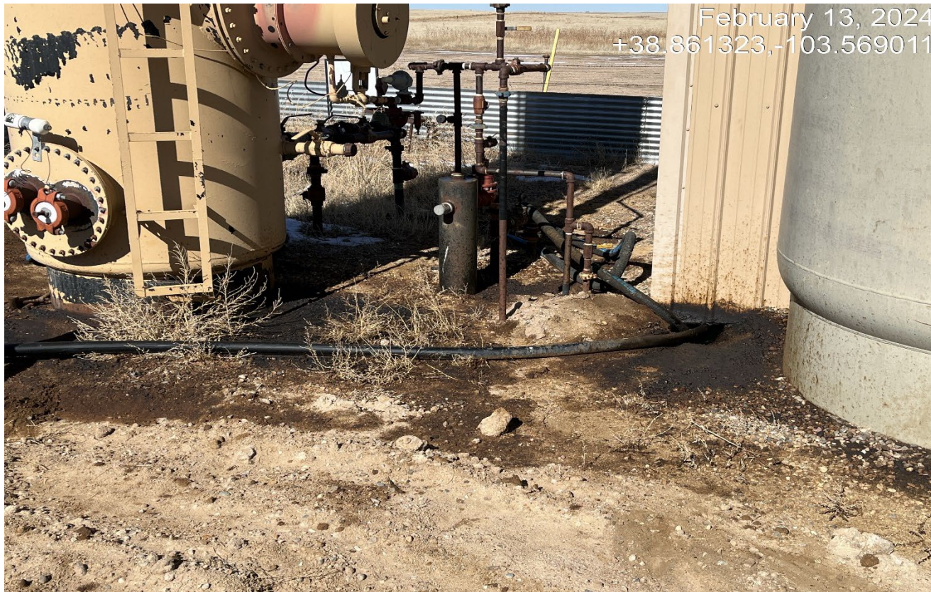
Photo 4. There are oil saturated soils around the treater that us be cleaned up.
