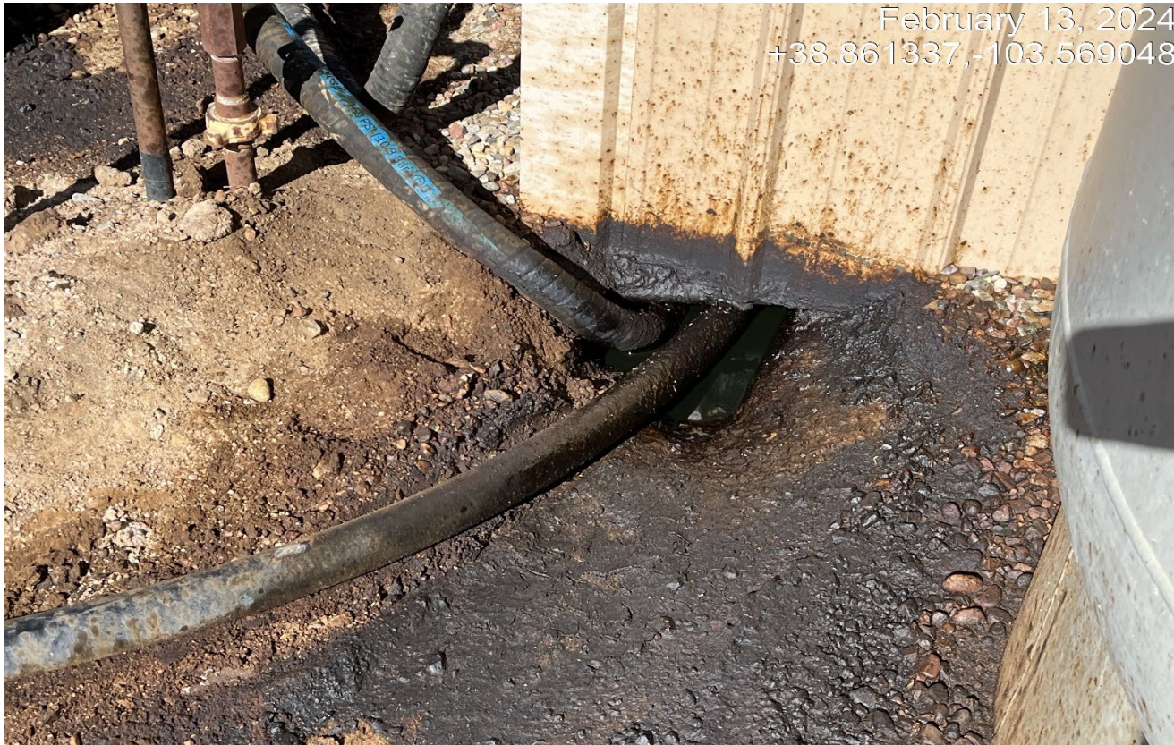
Photo 5. There is oil puddled up where the hoses go into the shed which indicates saturated soils and unknown amount of spill volume.
