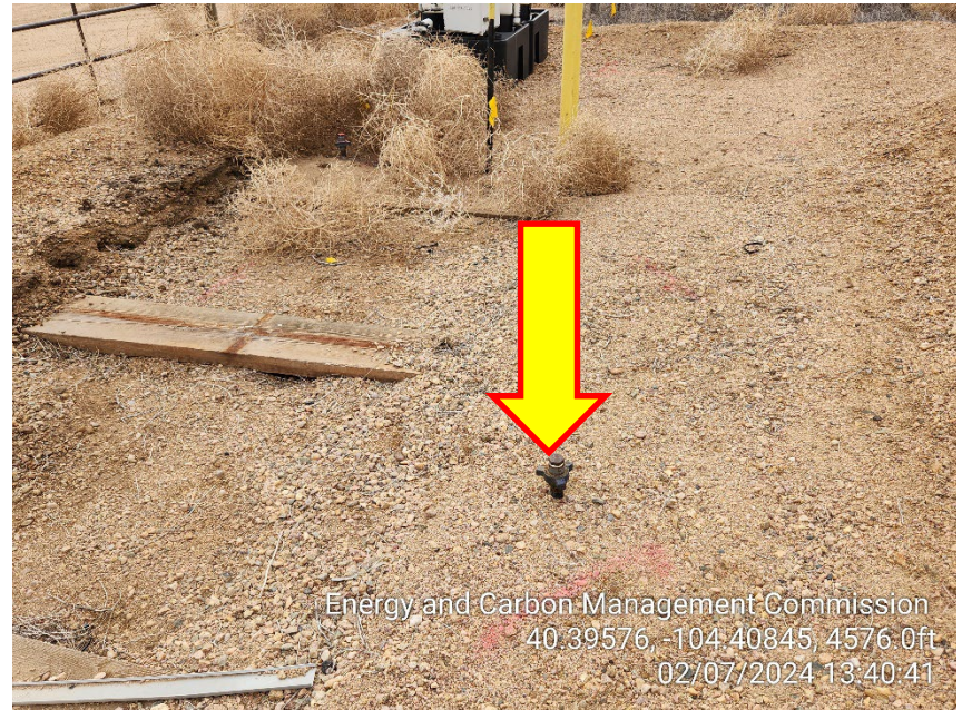
Photo 4 – Unmarked Riser
