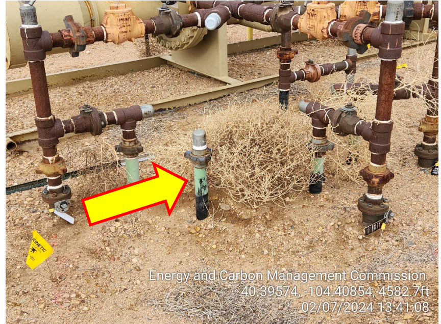
Photo 8 – Unmarked Riser
