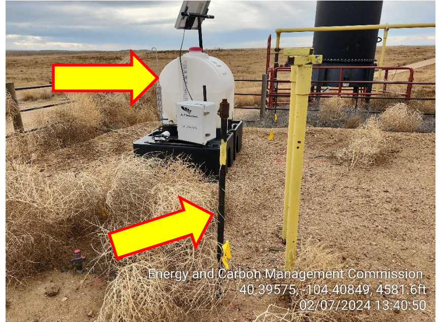
Photo 6 – Unmarked Riser and Unused Chemical Tank
