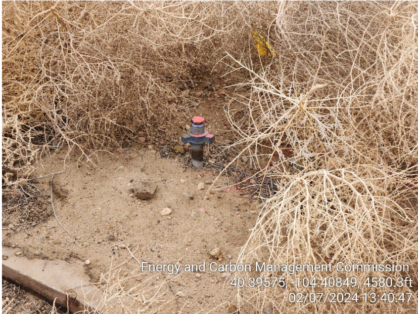
Photo 5 – Unmarked Riser and Tumbleweeds
