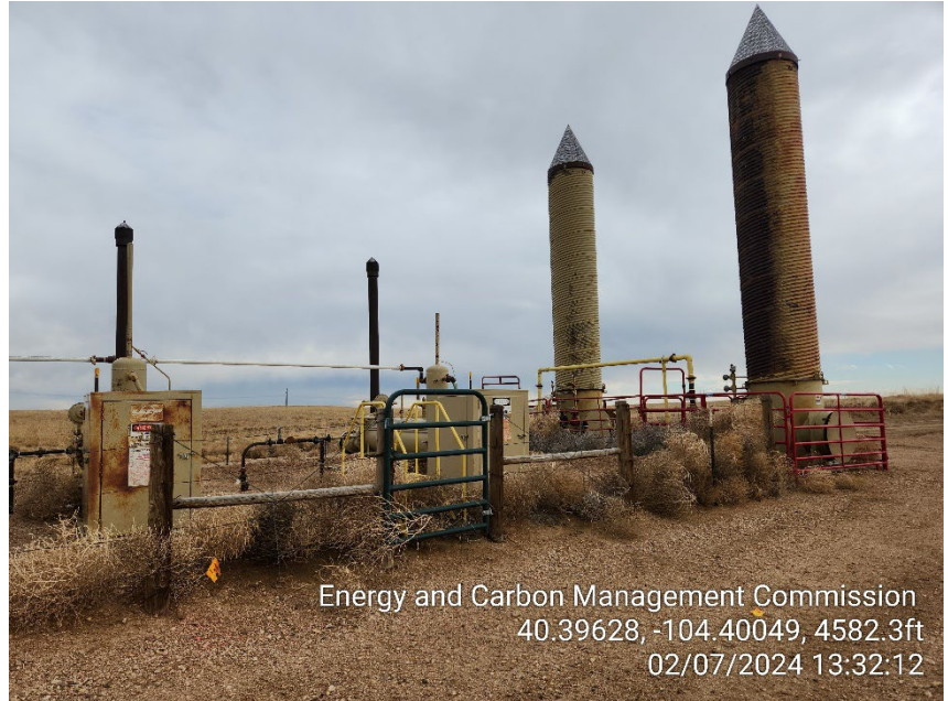
Photo 6 – Separators and ECDs
