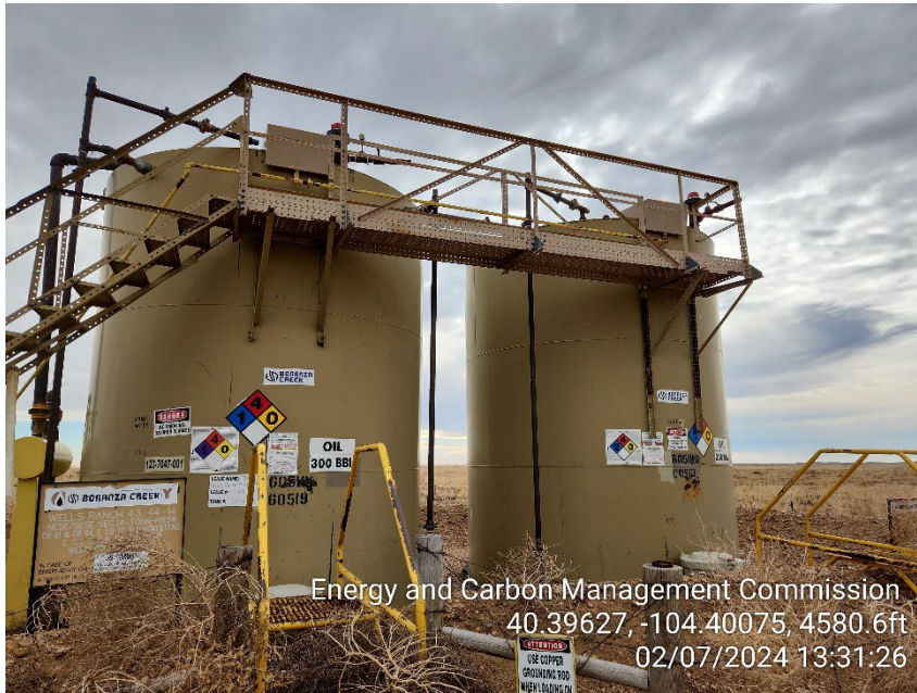
Photo 3 – Tank Battery
