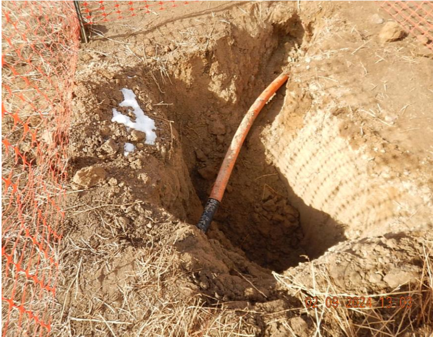
Off location flowline exposed in excavation; two pipe types/ colors joined via butt end poly fusion welding
