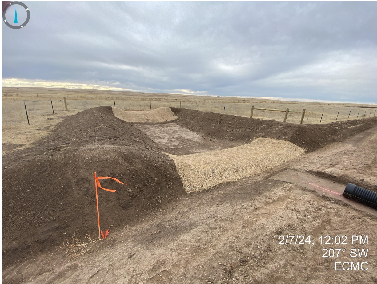
Photo 19. The southern sediment trap is still being constructed at the time of this inspection.
