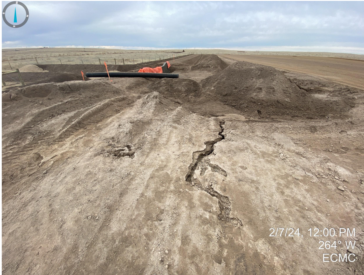
Photo 17. Erosion degradation occurring near the southern sediment trap.
