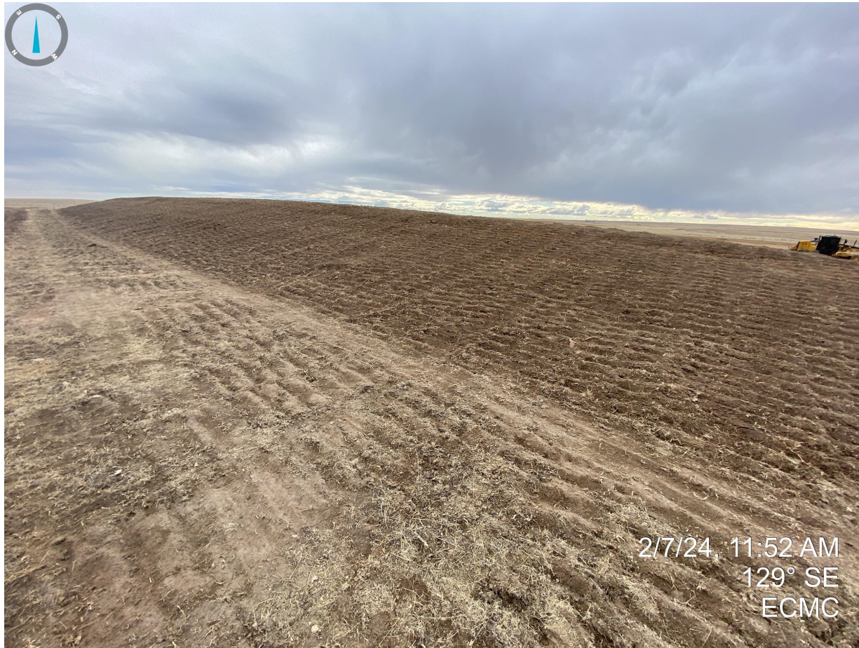
Photo 11. Northwest portion of the drilling pad topsoil stockpile. It appears the stockpile has been temporarily stabilized with evidence of equipment tracking.
