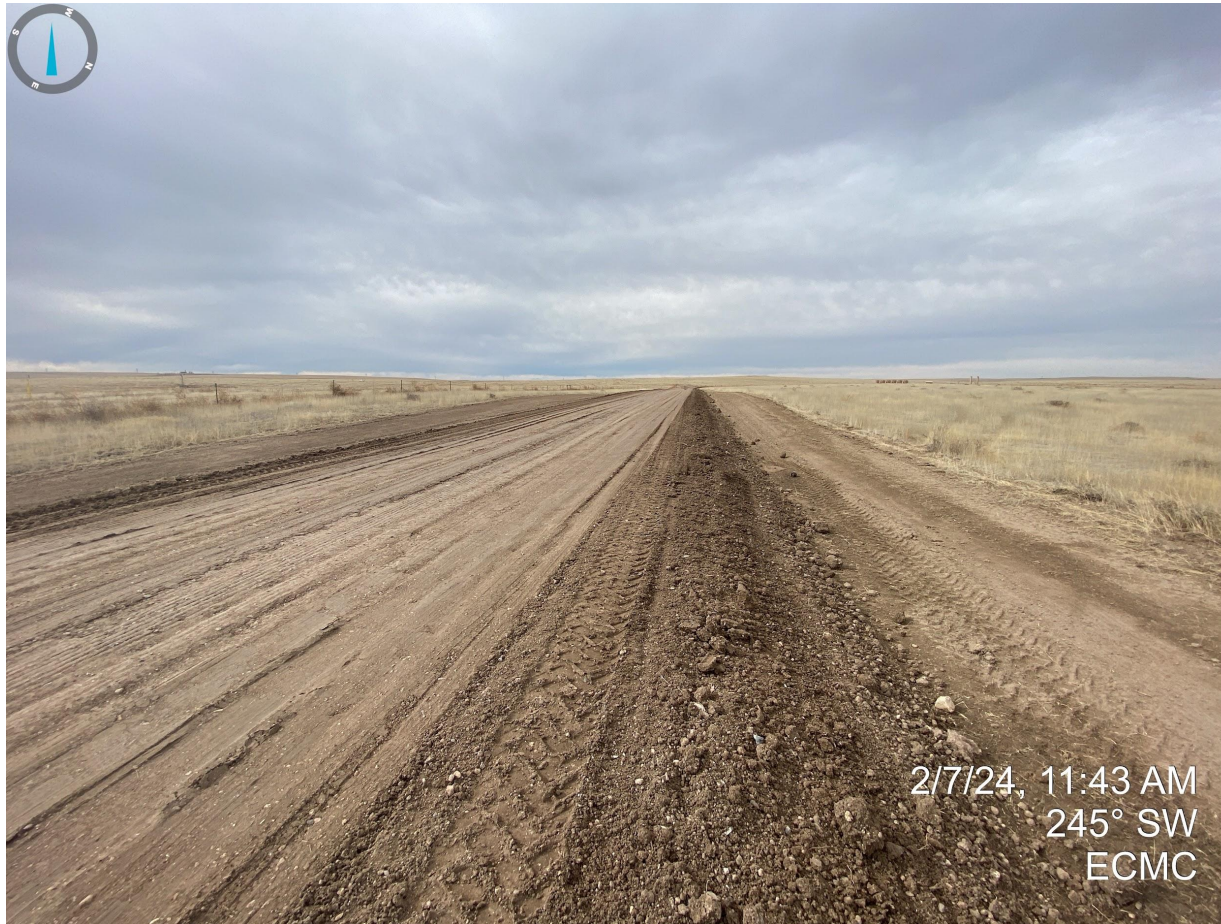
Photo 4. Taken from the middle portion (between the two culverts) of the access road. It doesn't appear that any topsoil has been salvaged from the access road since the previous inspection. It also appears that road base has been applied over existing topsoil.
