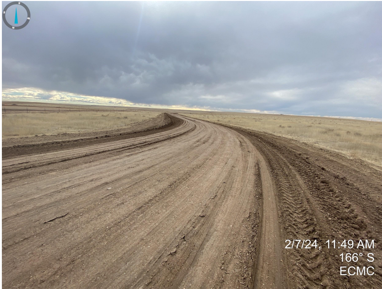
Photo 7. Taken near the entrance to the drilling pad and the access road. It doesn't appear that any topsoil has been salvaged from the access road since the previous inspection. It also appears that road base has been applied over existing topsoil.
