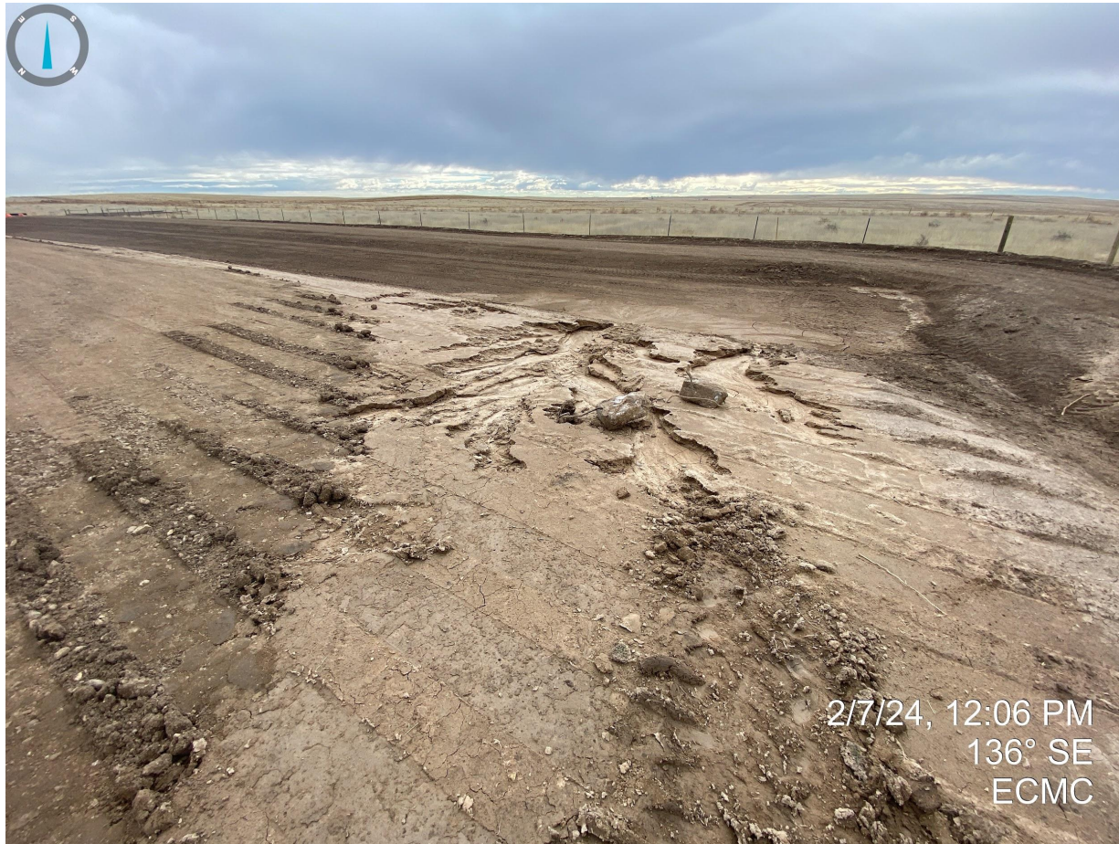
Photo 22. Erosion degradation and sediment transport observed on the southwest corner of the drilling pad.
