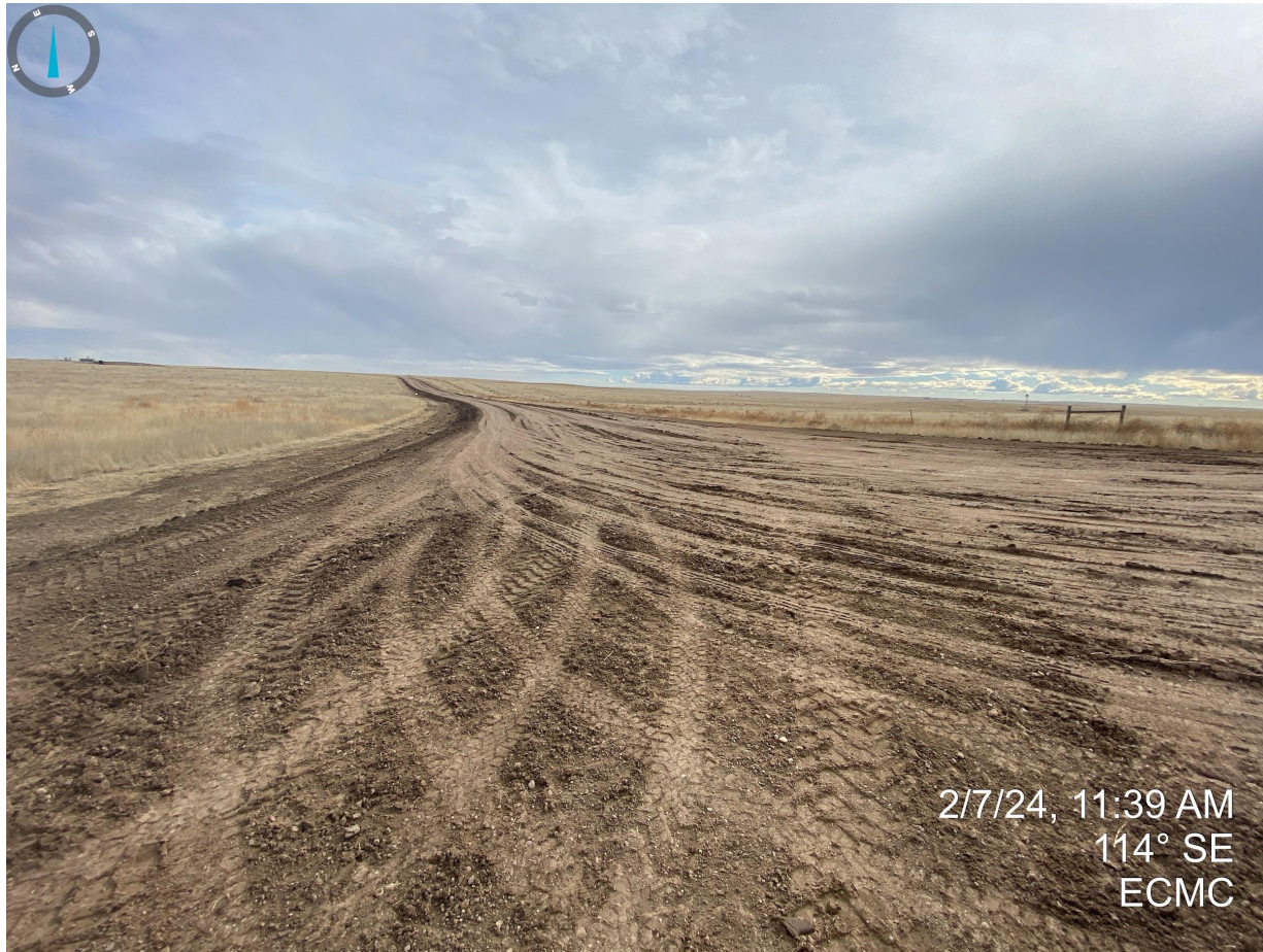
Photo 1. Taken from the start (west end) of the access road. It doesn't appear that any topsoil has been salvaged from the access road since the previous inspection. It also appears that road base has been applied over existing topsoil.
