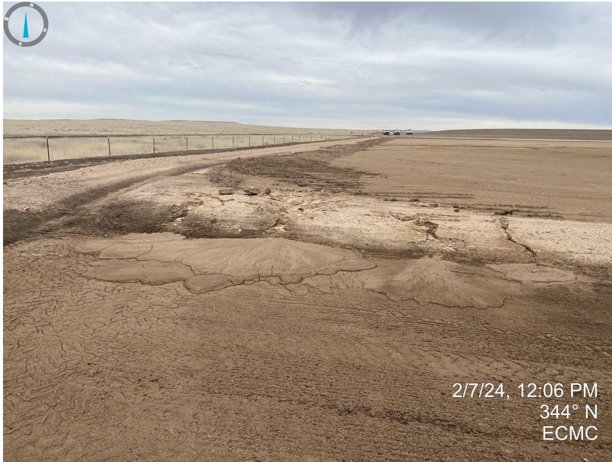
Photo 21. Erosion degradation and sediment transport observed on the southwest corner of the drilling pad.
