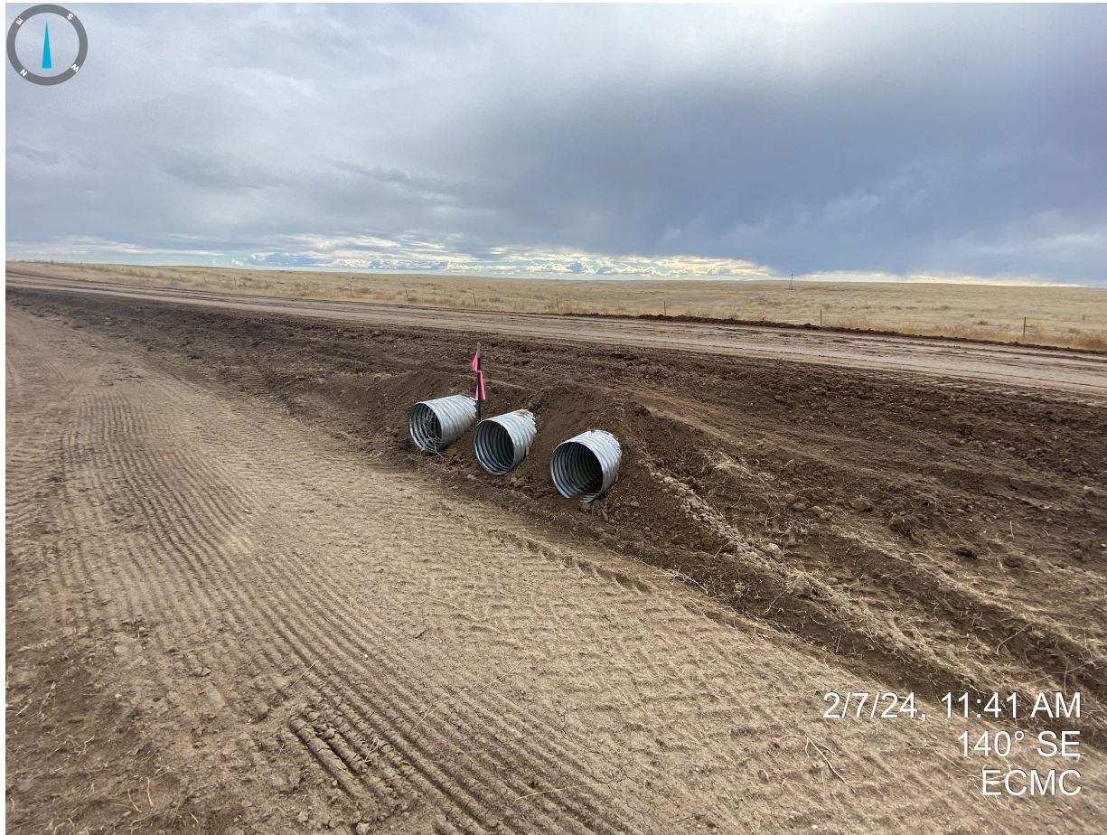
Photo 2. Taken near the west culvert crossing (north side). It doesn't appear any topsoil has been salvaged since the previous inspection and any topsoil used as fill at the culvert crossing has not been removed.
