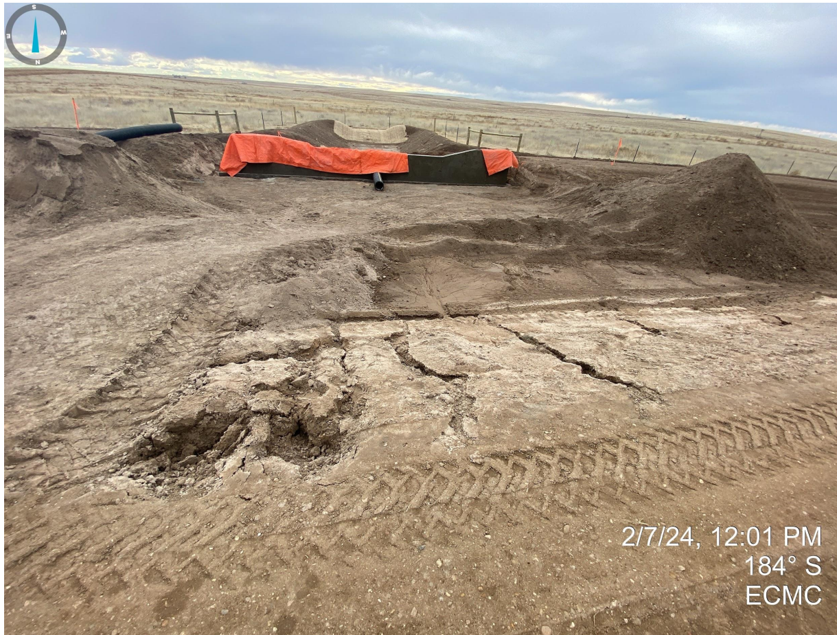
Photo 18. Erosion degradation occurring near the southern sediment trap. The southern sediment trap is still being constructed at the time of this inspection (pictured in background).
