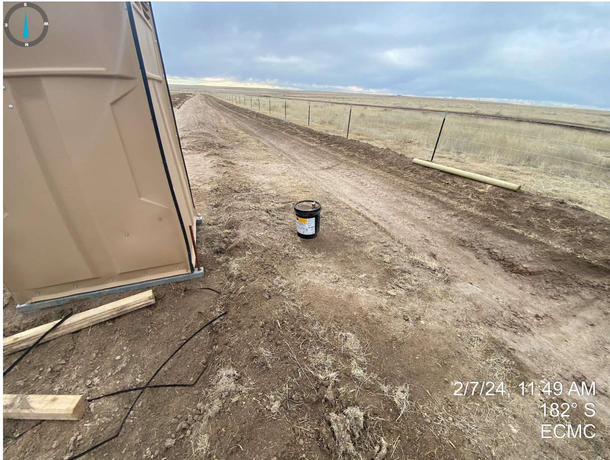
Photo 9. 5 gallon bucket of oil observed without any secondary containment, placed immediately adjacent to perimeter stormwater ditch.
