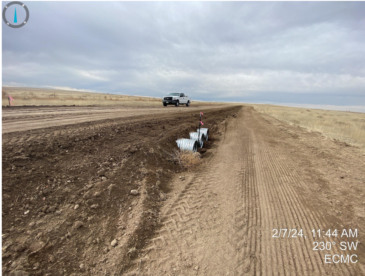
Photo 6. Taken near the west culvert crossing (north side). It doesn't appear any topsoil has been salvaged since the previous inspection and any topsoil used as fill at the culvert crossing has not been removed.
