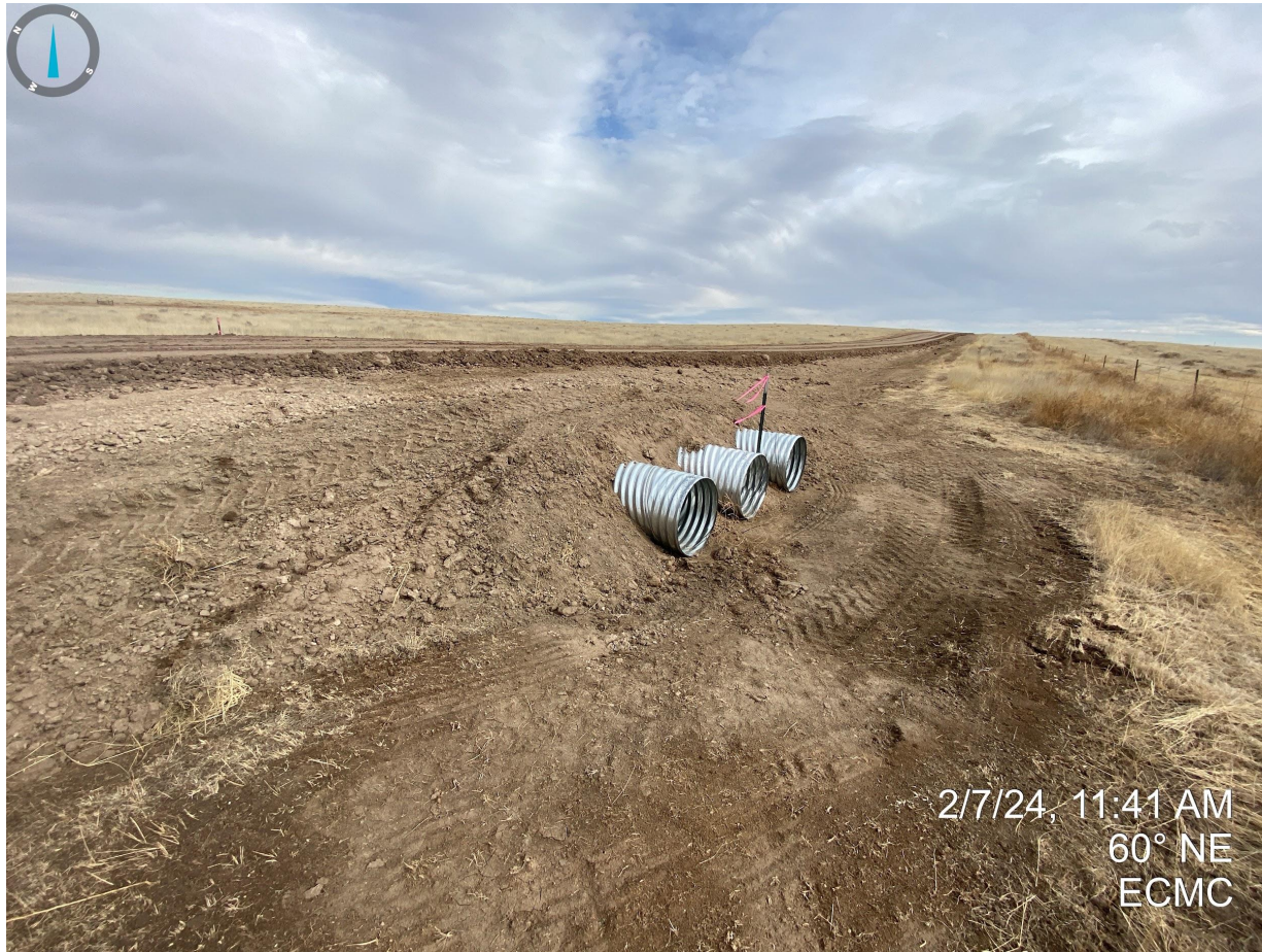
Photo 3. Taken near the west culvert crossing (south side). It doesn't appear any topsoil has been salvaged since the previous inspection and any topsoil used as fill at the culvert crossing has not been removed.
