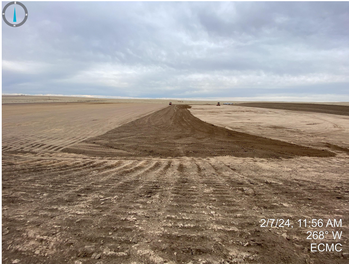
Photo 15. Taken from the eastern side of the location. Onsite crews were actively applying road base/armor to the drilling pad during this inspection.
