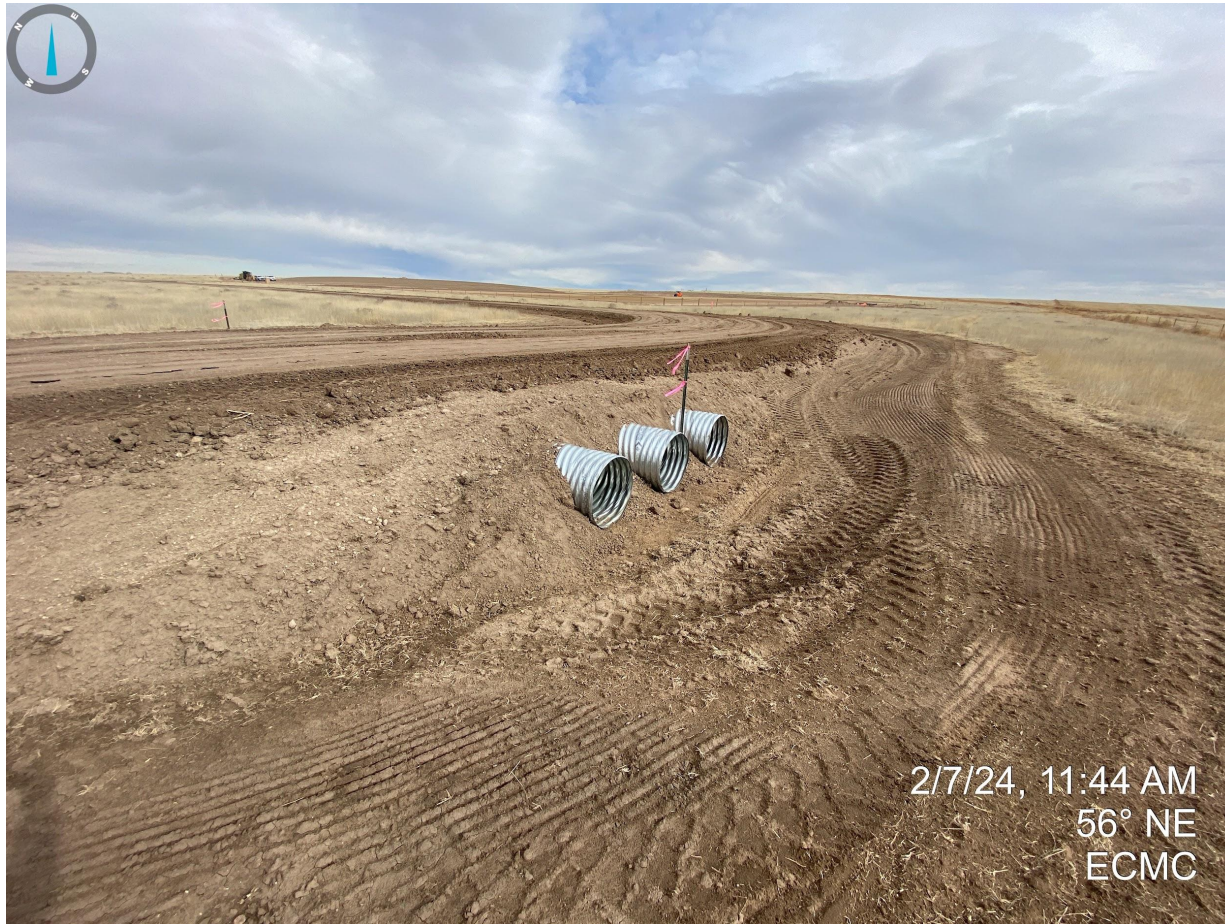
Photo 5. Taken near the east culvert crossing (south side). It doesn't appear any topsoil has been salvaged since the previous inspection and any topsoil used as fill at the culvert crossing has not been removed.
