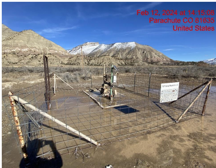
Wellhead/Site Degradation from Lack of Drainage – Photo #09196
