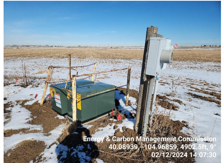
Photo 6 Electric panel, meter box and transformers.
