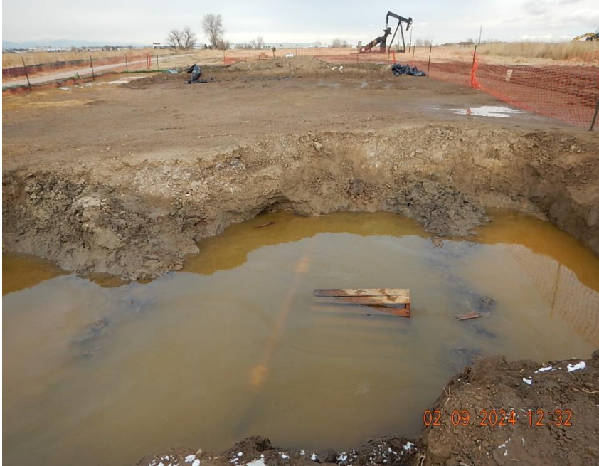
View of flowline pipe exposed in excavation; replacement section of fiberglass pipe is submerged under water/ fluids.
