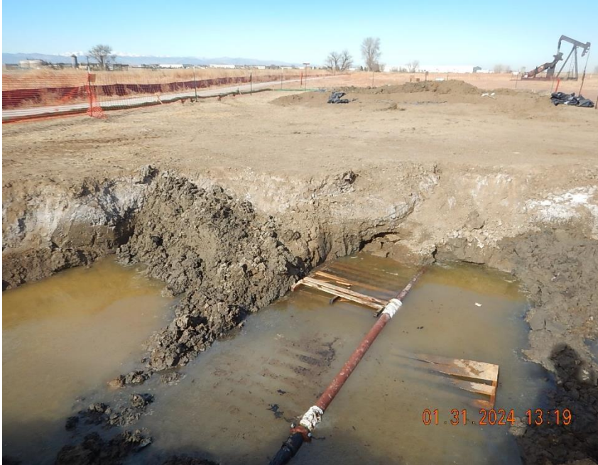
View of on location flowline pipe exposed in excavation; replacement section of 3" OD fiberglass pipe in area of failure.
