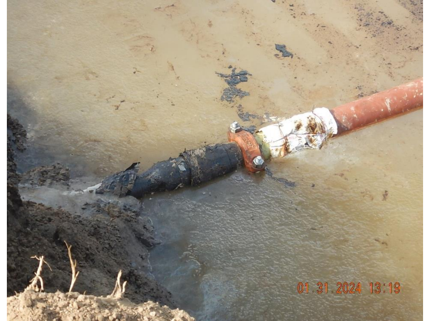
View of transitional fittings used to connect 3" OD fiberglass pipe to existing 2" carbon steel flowline pipe at south wall of excavation. Threaded fitting connections and a bolted clamp are being used; external pipe coating appears to be inadequate to protect from external and/ or thread corrosion.
