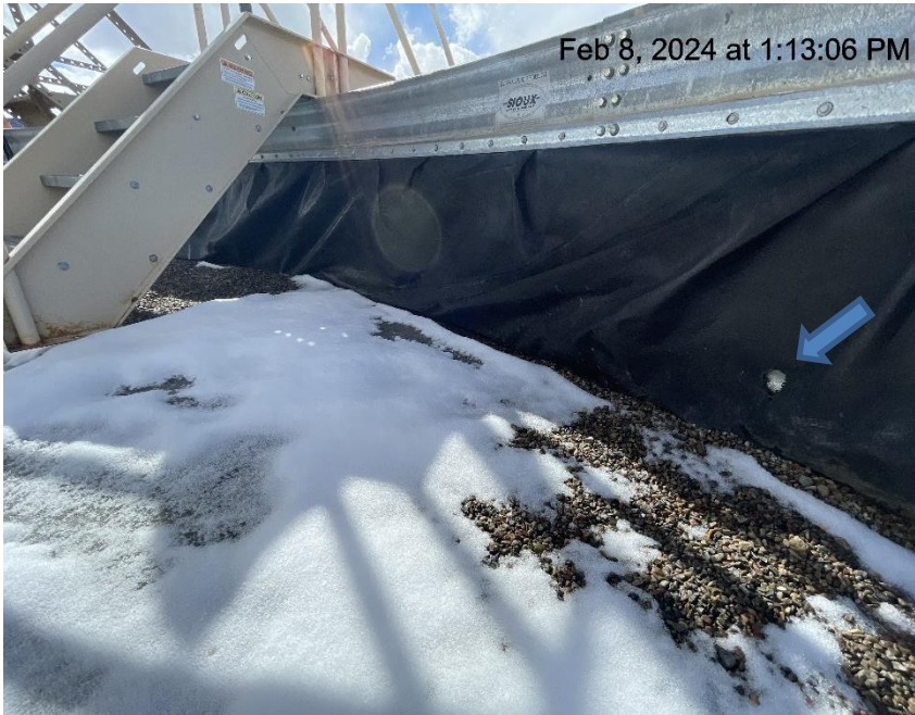
Photo # 6139 Hole in liner/liner needs maintenance
