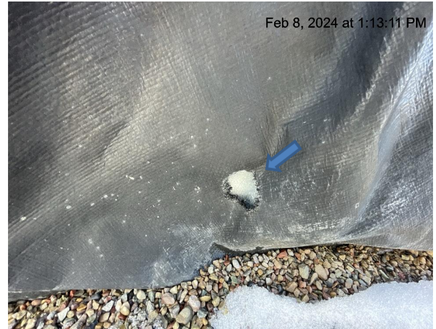
Photo # 6140 Hole in liner/liner needs maintenance
