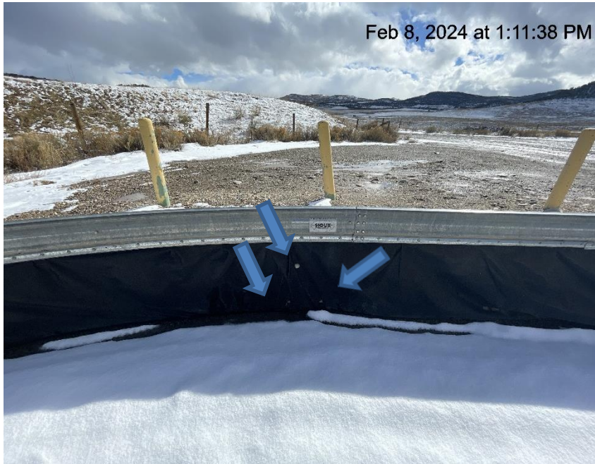
Photo # 6135 Holes in liner/liner needs maintenance
