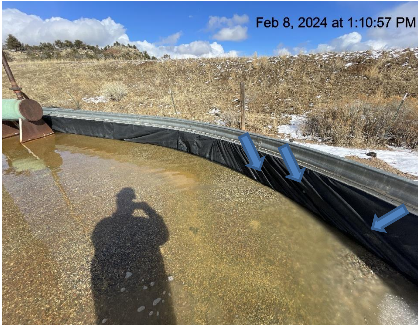
Photo # 6133 Holes in liner/liner needs maintenance
