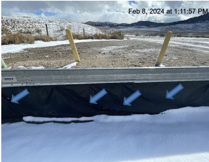
Photo # 6137 Holes in liner/liner needs maintenance
