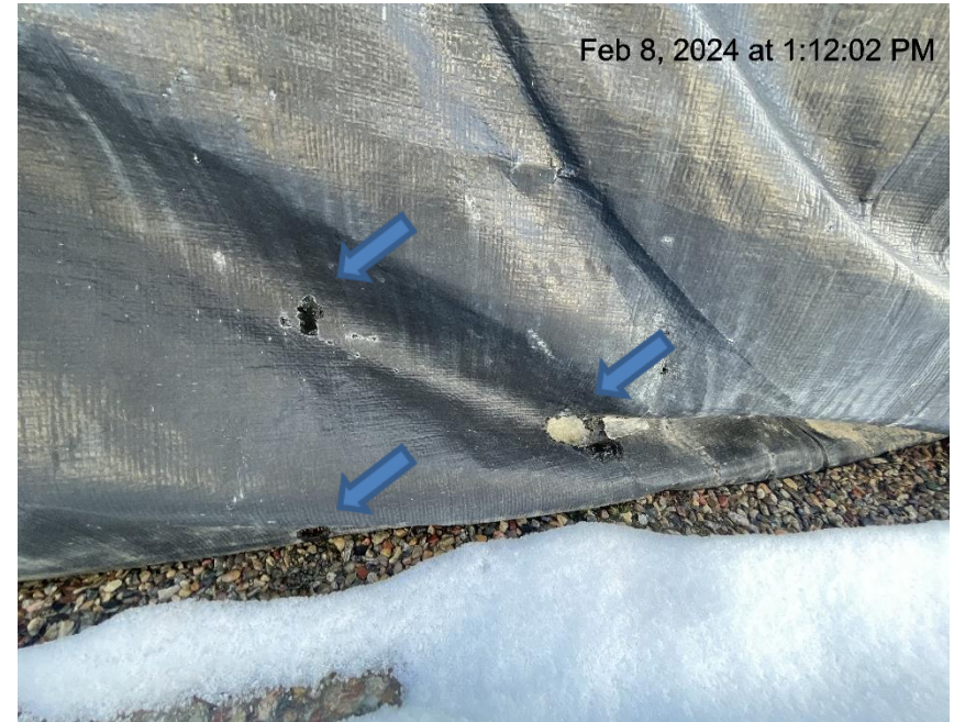
Photo # 6138 Holes in liner/liner needs maintenance
