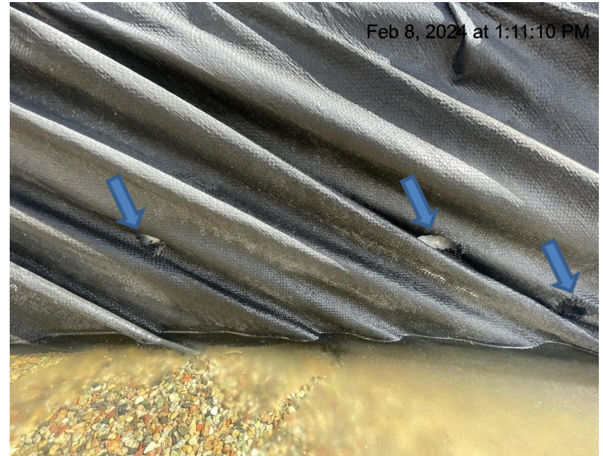
Photo # 6134 Holes in liner/liner needs maintenance
