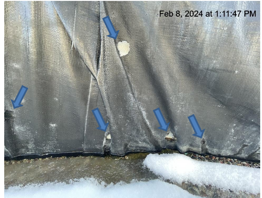
Photo # 6136 Holes in liner/liner needs maintenance
