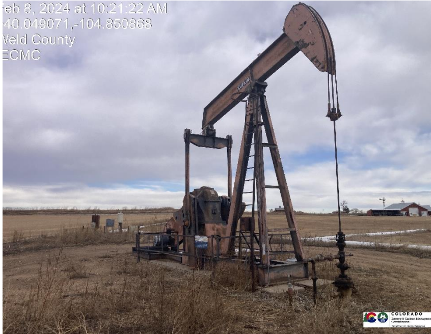
Pic 1 wellhead / pump jack
