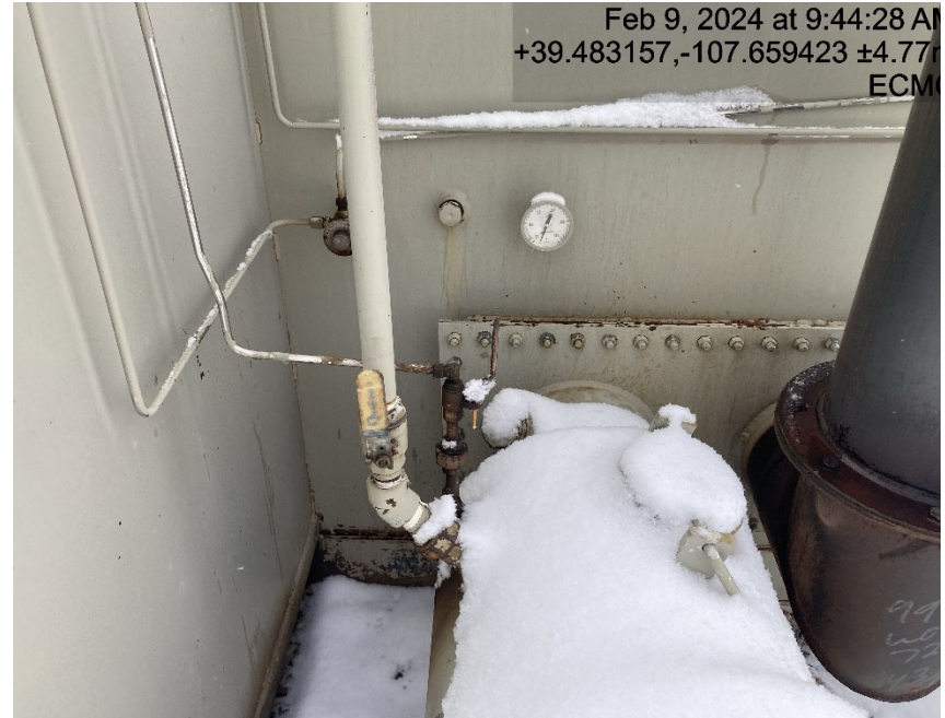
Valves open and gas running to burner, burner is not lit and venting gas.
