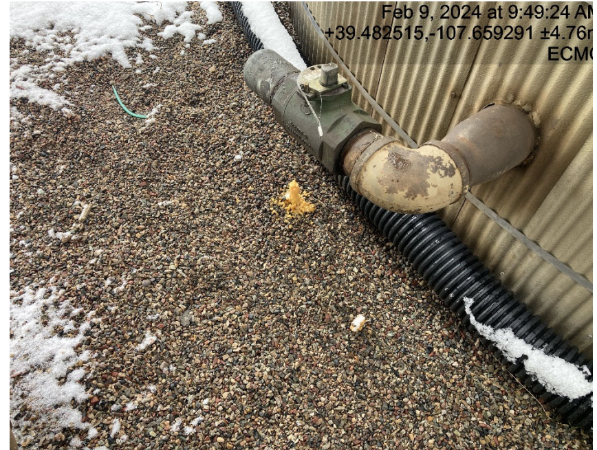
Valve leaking
