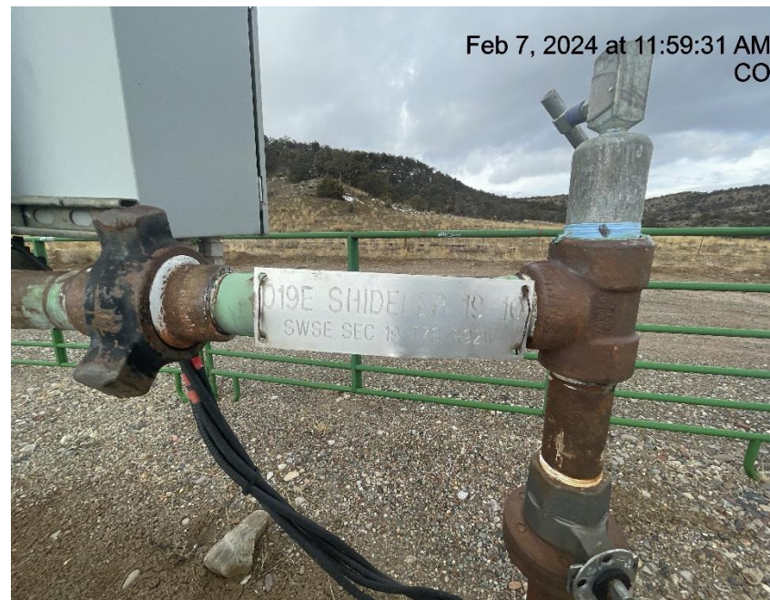
Photo # 5964 Wellheads lack required signage/signs missing required information
