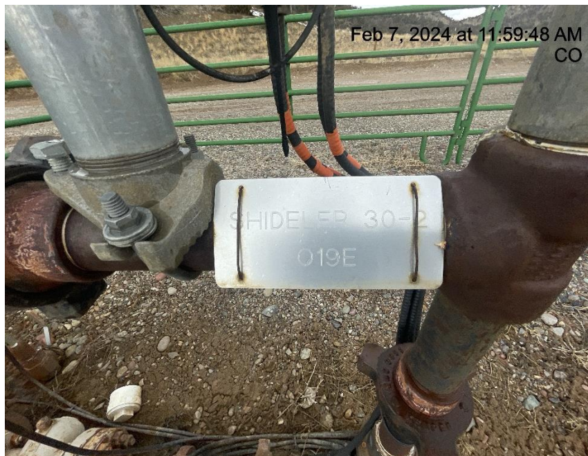
Photo # 5963 Wellheads lack required signage/signs missing required information
