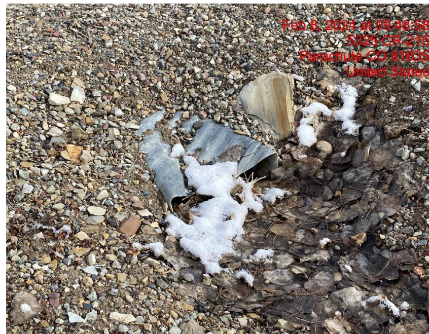
Damaged Culvert – Photo #09158
