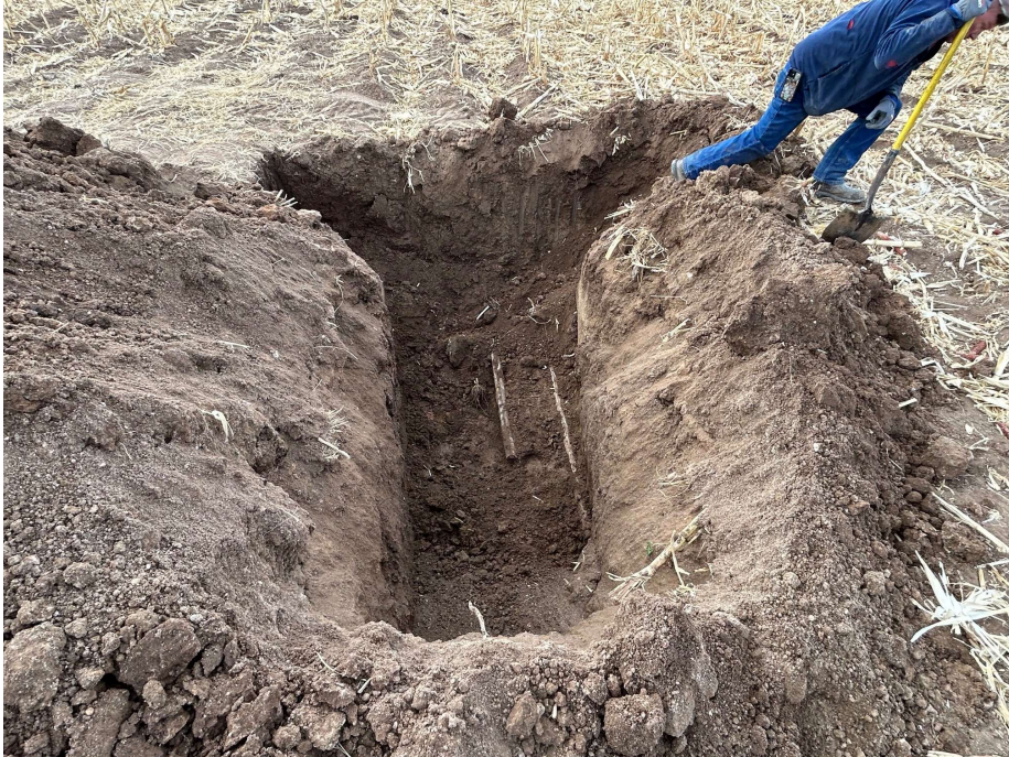
Well 35-4 Wellhead flowline ends after risers removed. Soil sample collected from bottom of excavation under flowlines.
