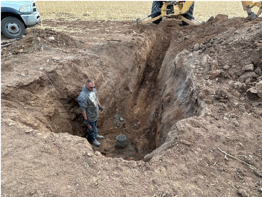
Well 35-4 Wellhead excavation.
