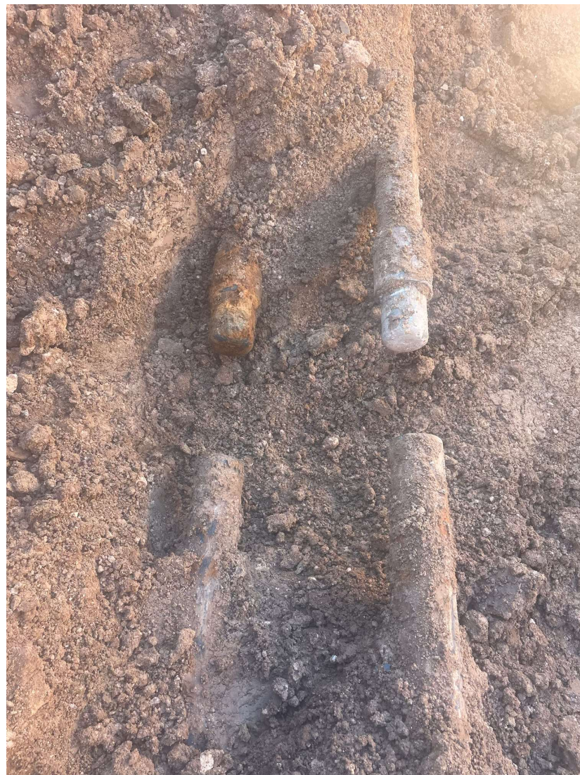
Flowline Cut & Cap Excavation. Mixed fluid located on the right and Natural gas on the left. Soil sample collected below cut area.
