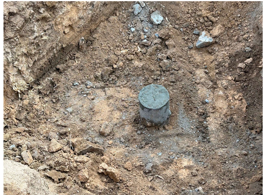
Well 35-4 Wellhead cemented to top and ready to have a steel plate welded in place. Soil sample collected adjacent to casing.
