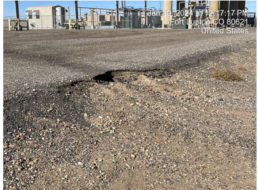
Photo 8. Photo taken of stormwater erosion on well pad perimeter. Photo taken facing northeast.
