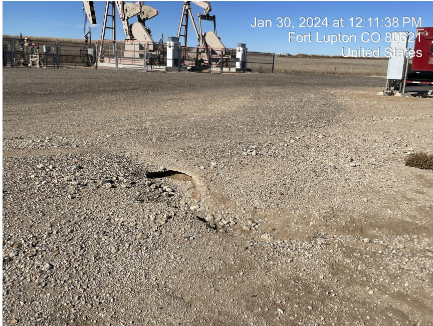
Photo 7. Photo taken of stormwater erosion on well pad perimeter. Photo taken facing north
