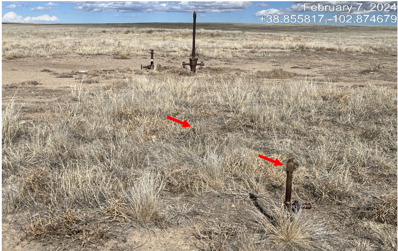
Photo 2. There is a metal bar and unused riser that is unmarked and unused.
