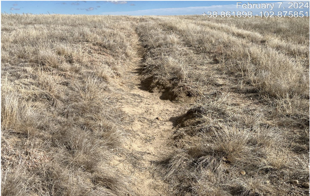
Photo 2. There is an erosion channel along the road closer to the location that needs to be repaired.
