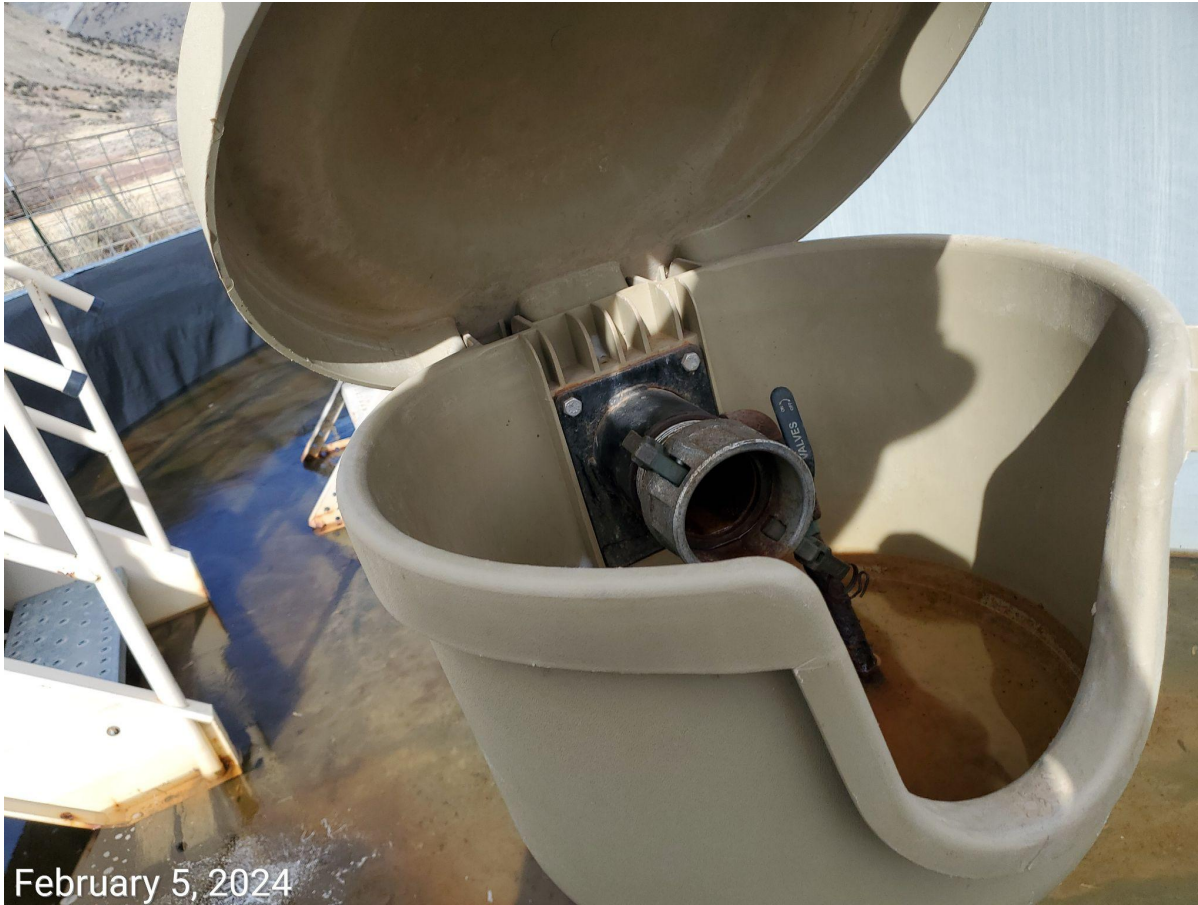
Photo 2: Line at tank not capped/plugged.
