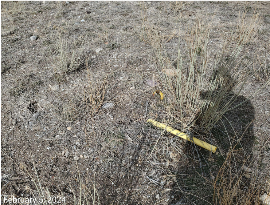
Photo 4: Anchors missing required marking pursuant to Rules 1003.a and 603.j.
